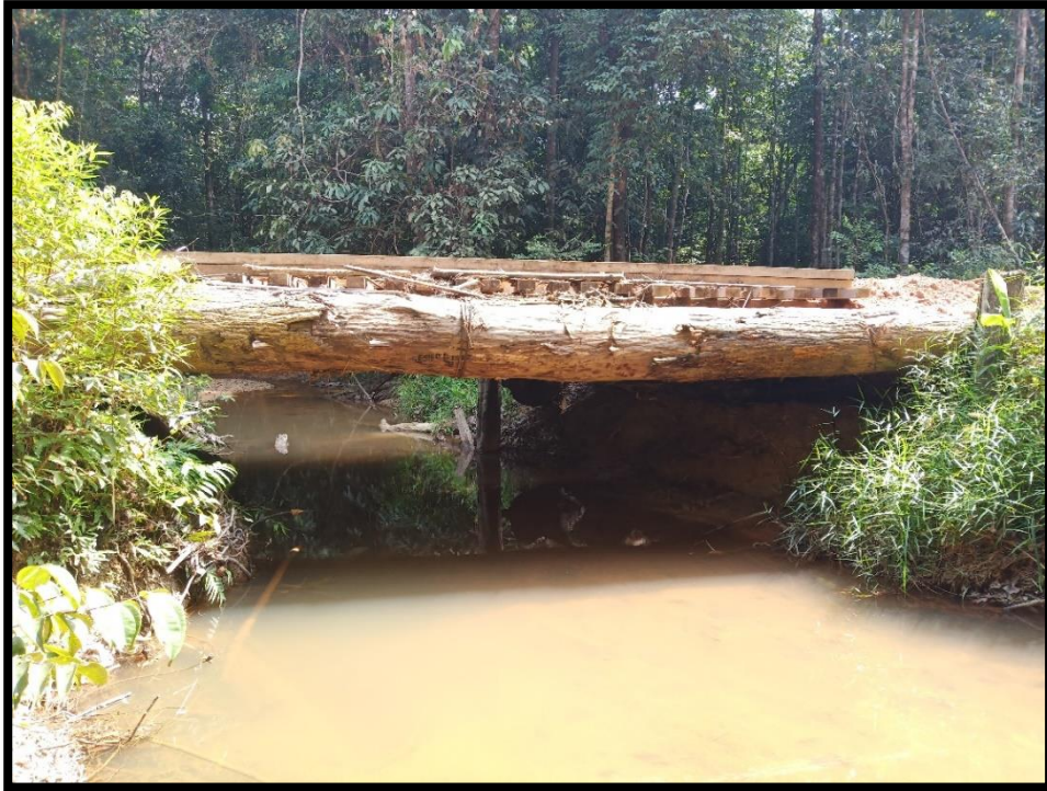
Plate 2.2 Permanent log girder bridge requiring heavy installation equipment, illustrating deployment inflexibility inherent to fixed infrastructure solutions.
