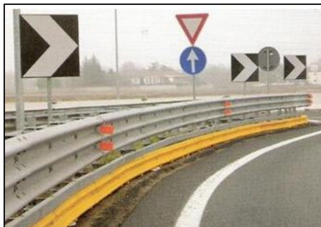
Figure 2.1 Spanish Guardrail That Meets Motorcycle Safety Standards (Nicol et al., 2012)
