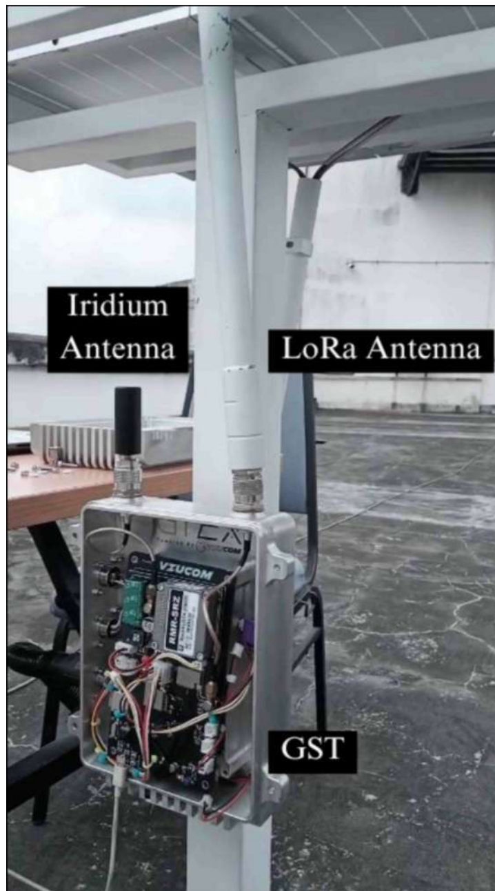
Figure 4.9 On-Site Testing of GST System
