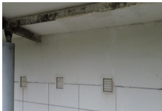
Figure 1 Mould growth from an image taken by UAV
