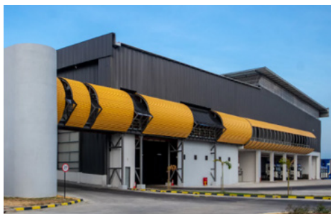
Figure 13. Attached Tubular Pathway to the Building
