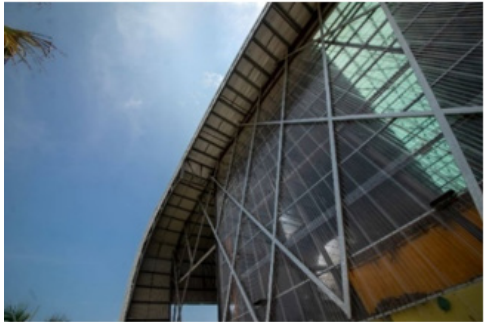
Figure 9. Glass Façade with Floor-to-ceiling Transparent Material Panels Source: SteelPedia-Batu Maung Waste Transfer Station, 2019
