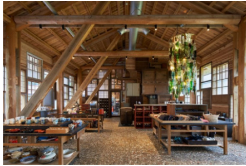
Figure 5. The Exposed Timber Structure
