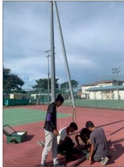
Figure 2: Repair of a Spotlight
