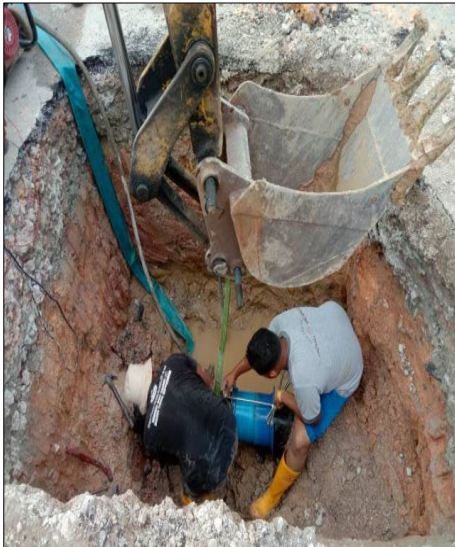
Figure 3: Repair of a Leaking Water Pipe
