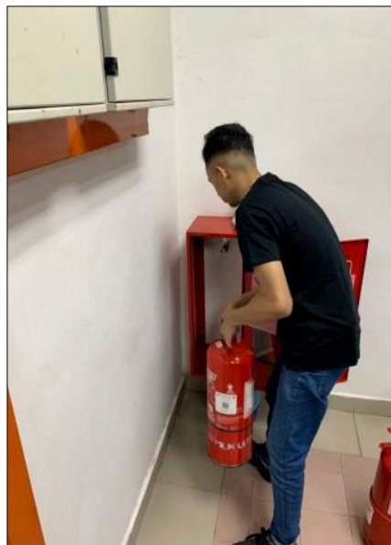
Figure 6: Fire Extinguisher Replacement
