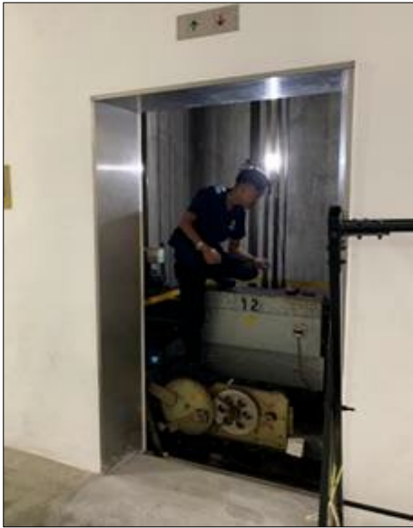
Figure 1: Repair of a Lift
