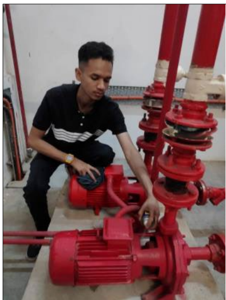
Figure 5: Fire Hydrant Inspection
