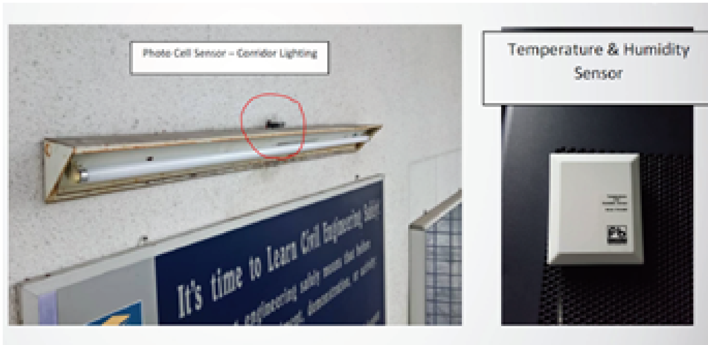
Smart Building Installation of photocell sensor at Engineering Complex
