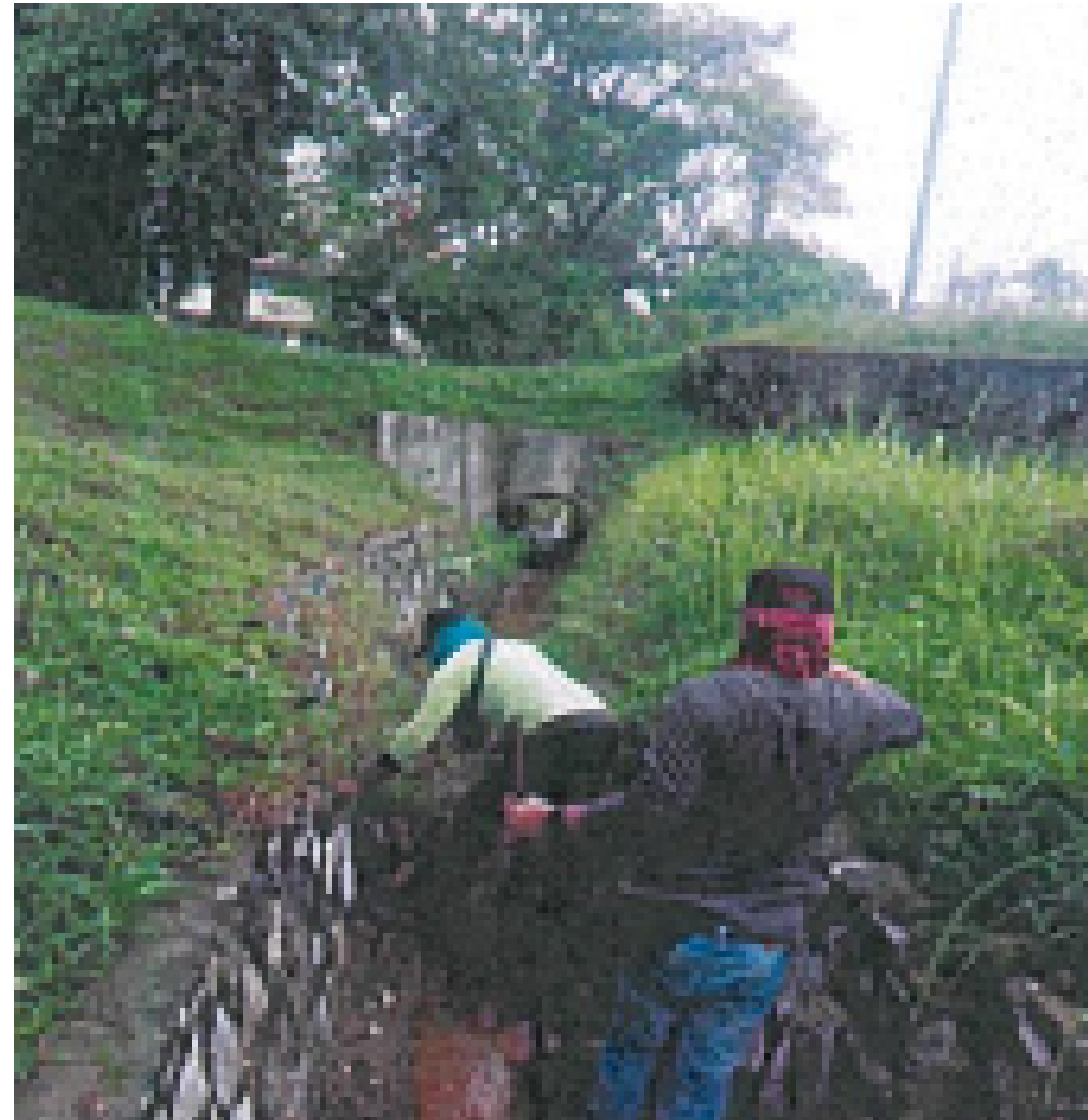
Monsun Drain Cleaning Routine Activities
