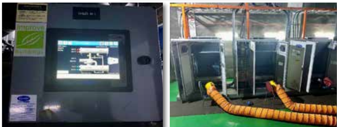
Figure 2.5: Replacement of four RT water-cooled chillers is the major project for energy saving at the Engineering Complex
