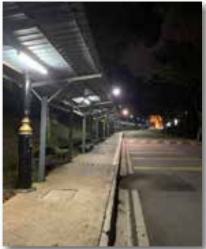
Figure 5.9: Well-lit and mostly covered path at night with speed humps strategically placed
