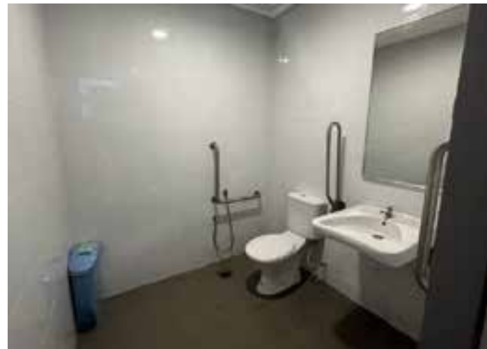
Figure 1.10: Designated toilet for disabled and special needs at Dewan Agong Tuanku Canselor, UiTM Shah Alam
