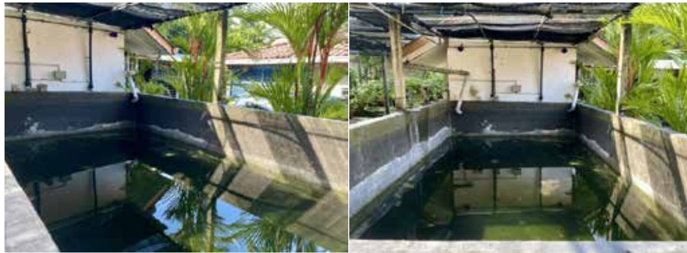
Figure 4.5: Rainwater being collected in the detention pond before being used for irrigation purposes
