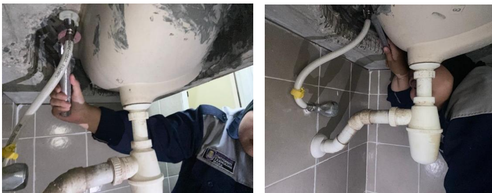
Figure 2 Comparison of wrench used in confined space: (left) modified wrench; (right) conventional wrench.
