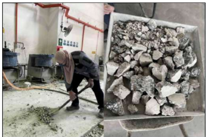
Figure 3.11 Recycled Concrete Aggregate Once Crushed (Big Size)
