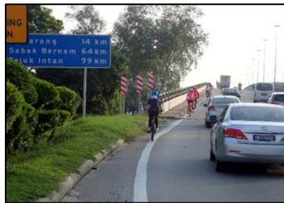
Figure 1. Overview of the Kuala Selangor Bridge approach.
