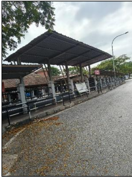
Fig. 3. Covered Walkway at SK Seksyen 7
