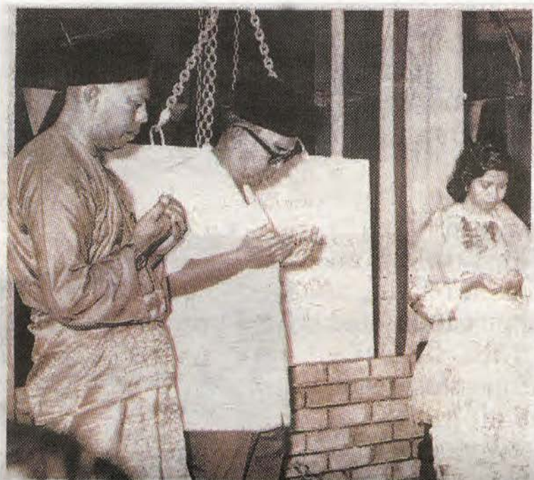
Tun Abdul Razak (second from left) reciting a prayer at the laying of the foundation stone ceremony at Rida headquarters building in Kuala Lumpur on June 6, 1965.
