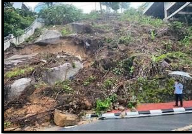
Figure 2. Landslide at Tanjung Bungah
