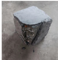
(f) Mortar (After)
