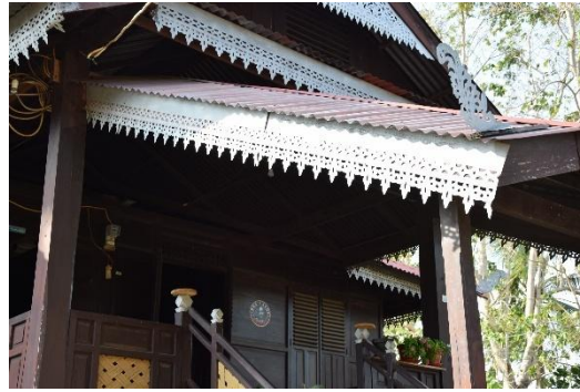
Pict.13. Full Ornament in the end roof Photographer : Andi Abidah 2015
