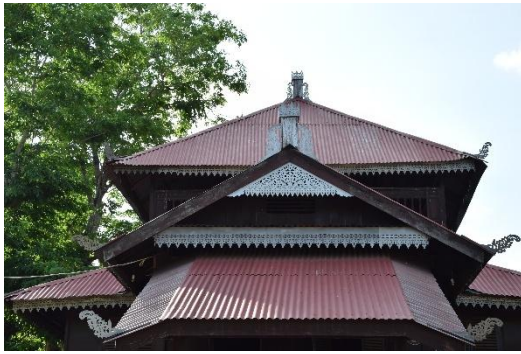
Pict 12. The roof did not apply saddle roof Photographer : Andi Abidah 2015
