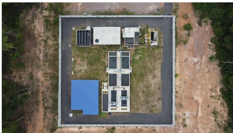
Figure 3. Top view of aeration pond in UiTM Segamat Campus
