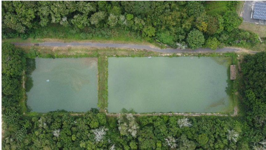
Figure 2. Top view of oxidation pond in UiTM Segamat Campus
