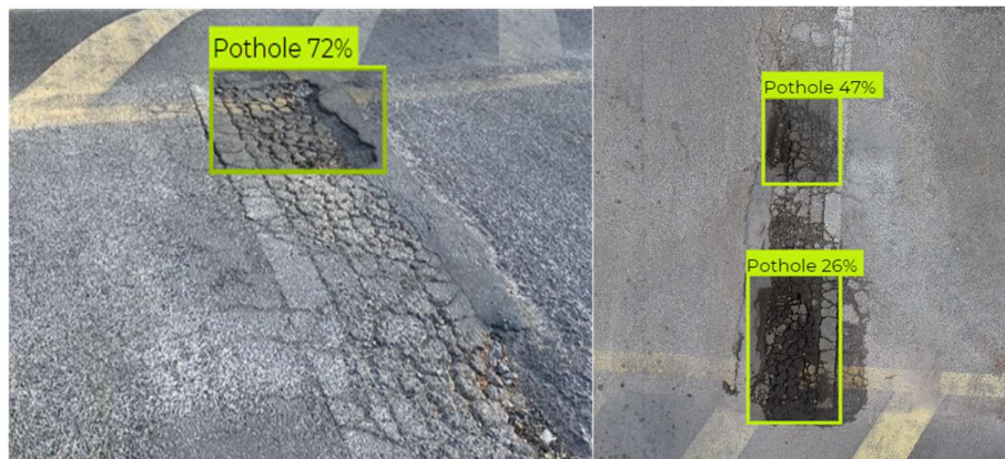
Figure 5: Result 2 pothole detection on camera image and orthophoto
