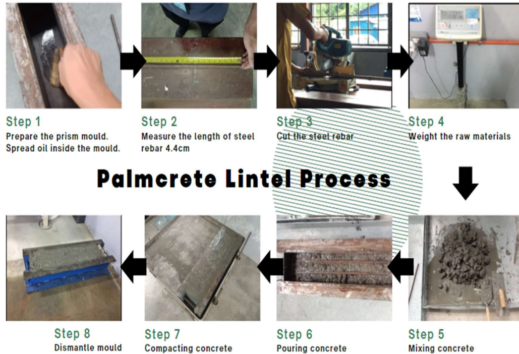
Figure 2.1 Process of Palcrete lintel
