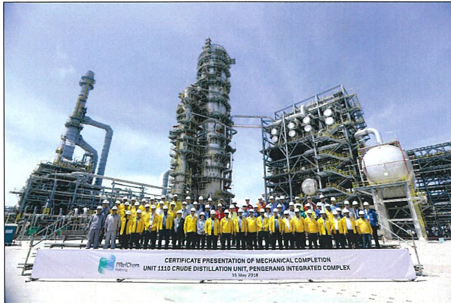
Figure 2.1.1 (b): The completion plant of PRefChem
