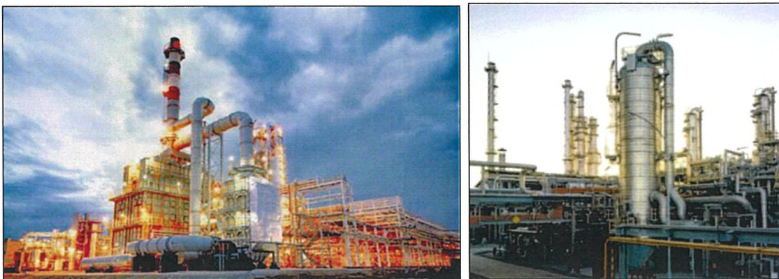
Figure 5.1.3 (b) State-of-the-art Lummus Technology and High-Efficiency trays in distillation columns
