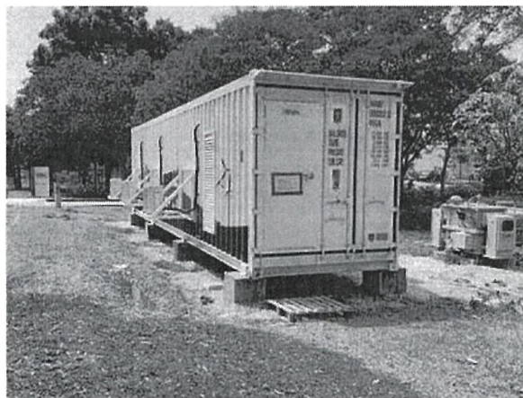
Figure 8: Battery Energy Storage System
