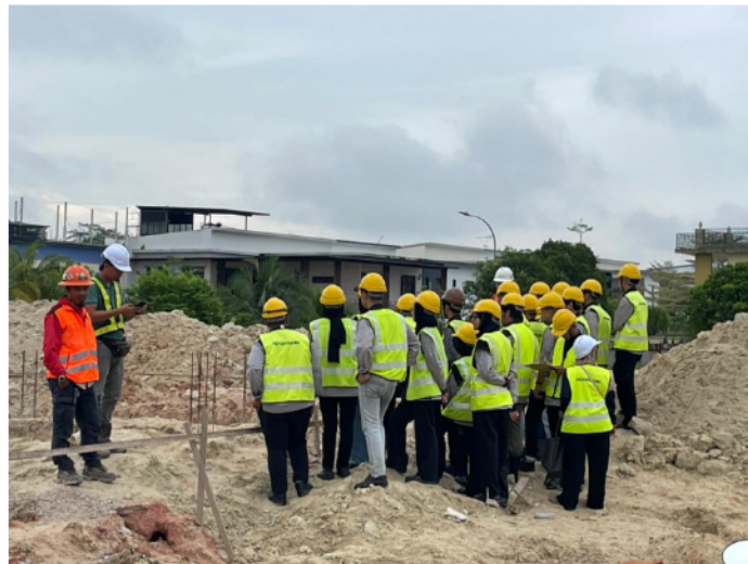
Fig. 3 Students observing the Excavation work.
