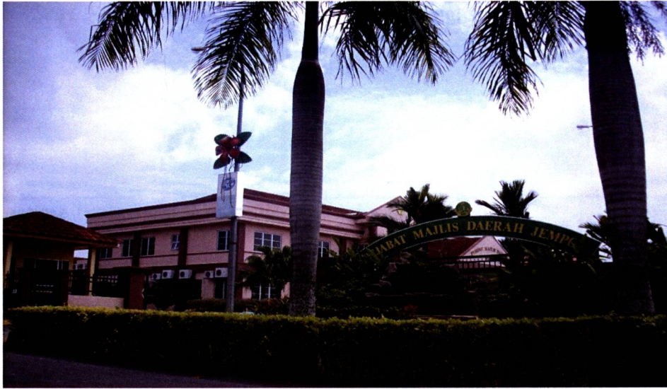
Figure 1.2 View of Jempol District Council
