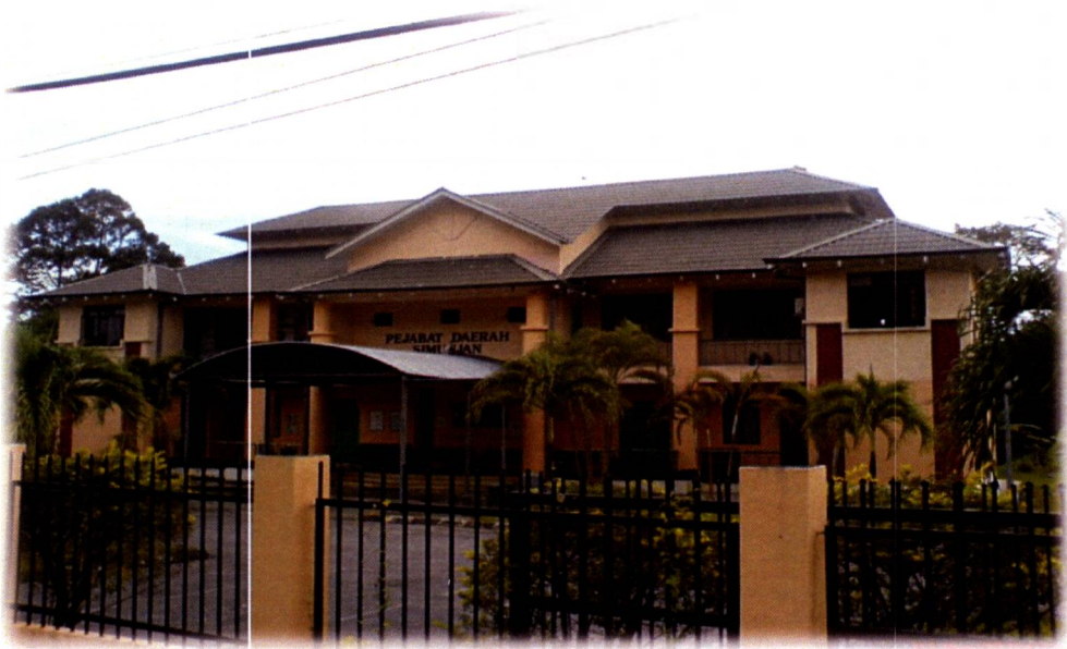
Figure 1.1 Simunjan District Office
