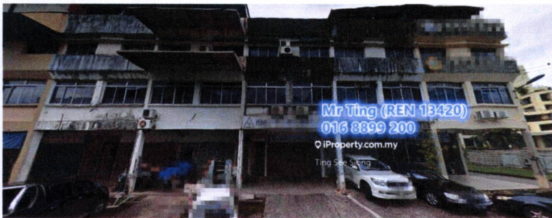
Figure 5.1.2. Dream Cake House Building
