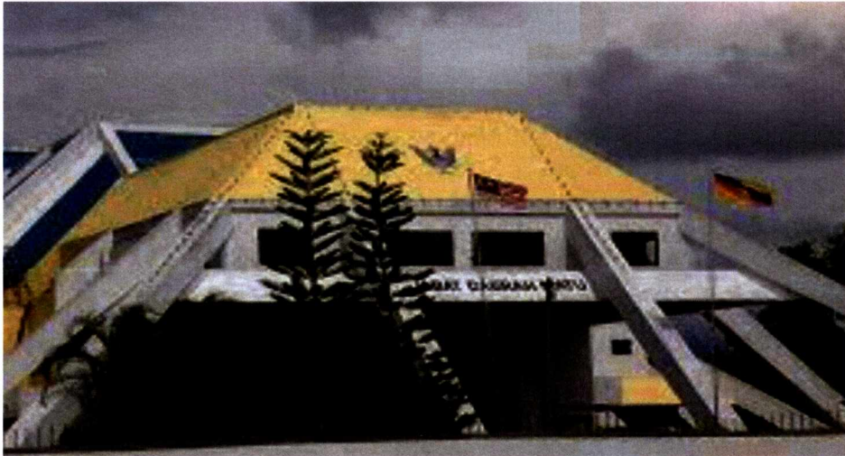
Figure 1.1 Matu District Office
