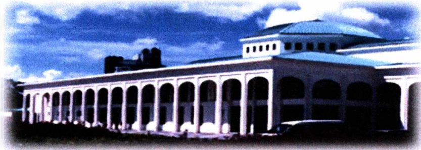
Figure 1: State Library Building: ( Pustaka Negeri Sarawak )
