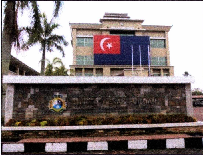
Picture 1.1.2: The main entrance of Pontian District Council
