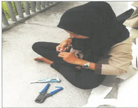
Figure 14: Patching Network Cable
