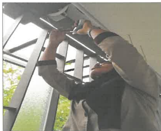
Figure 15: Installing Network Cable
