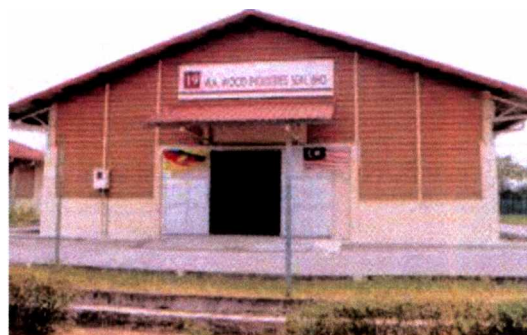
Figures 2.11 Site Visit to Kompleks Industri Perabot
