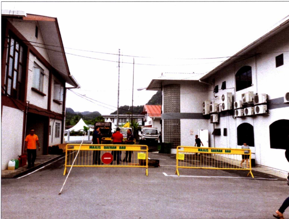
Figure 1.1 Bau District Council back view
