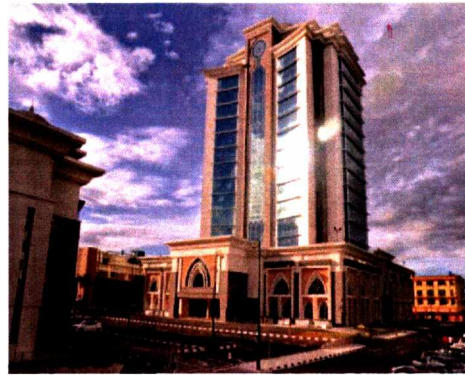
Figure 1.4: Resident and District Building (19 August 2015-Present)
