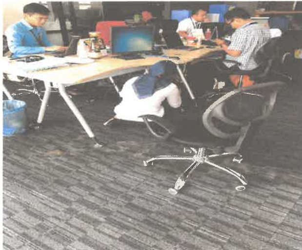
Figure 10: Trainee Ensuring All Cables Were Sort and Arranged Tidy
