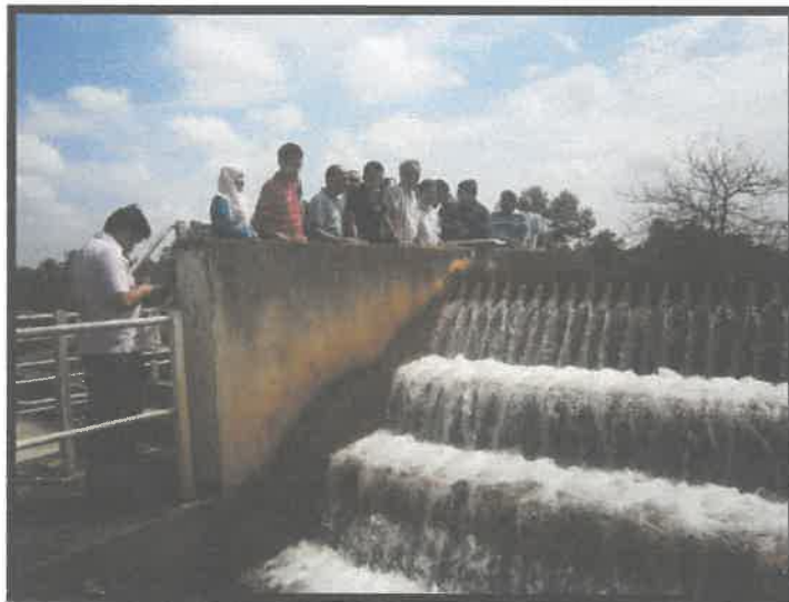
Figure 3.24: Water Treatment Plant (WTP) Chicha
