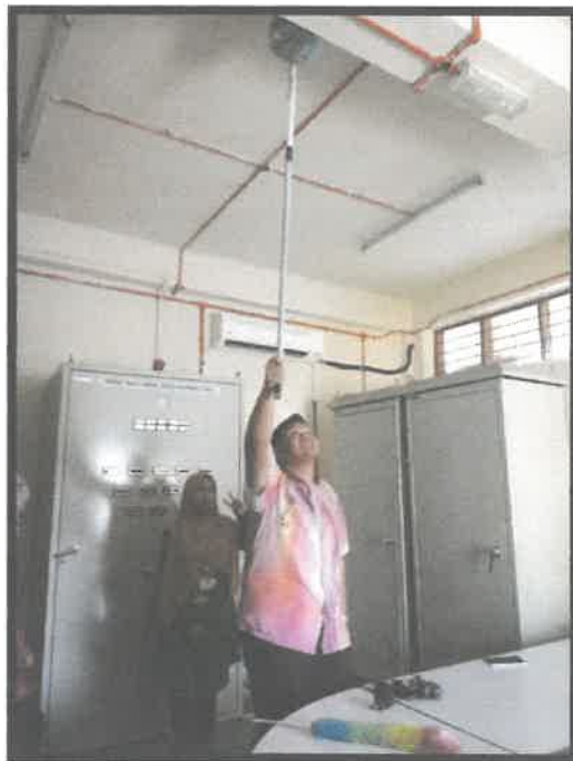
Figure 3.25: Housekeeping at WTP Kg. Puteh
