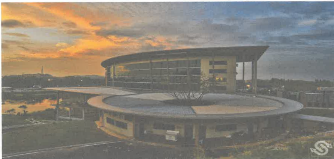
Figure 1: The building of Pustaka Raja Tun Uda
