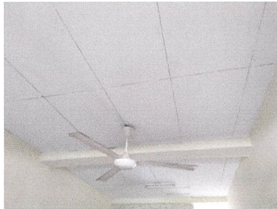
Figure 3.17: completed ceiling works
