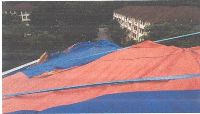
Figure 3.4: Temporary covering for roof structure
