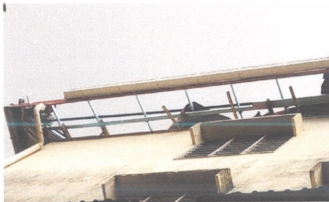
Figure 3.11: Installation of gutter
