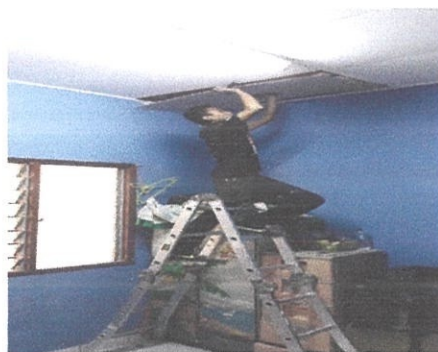
Figure 3.13: Dismantle existing ceiling structure.
