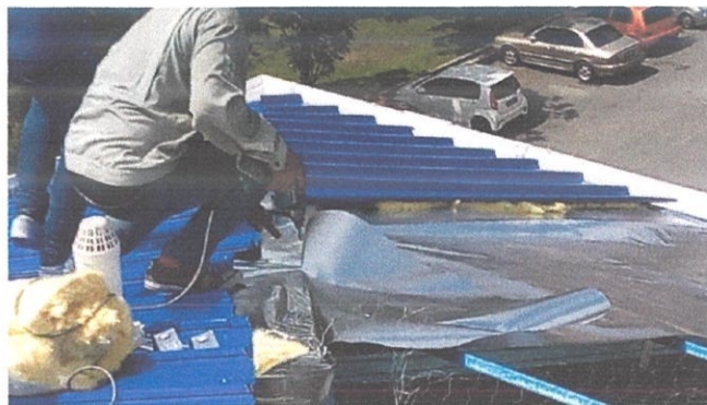
Figure 3.8: Installation of Aluminium Foil
