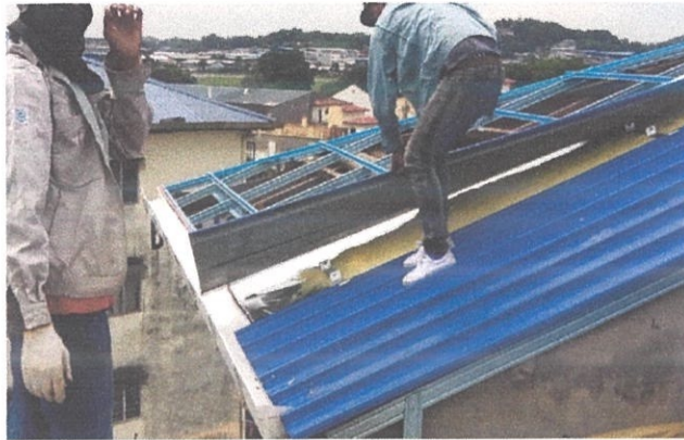
Figure 3.10: Installation of Metal covering
