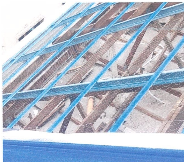
Figure 3.7: Installation of wire netting
