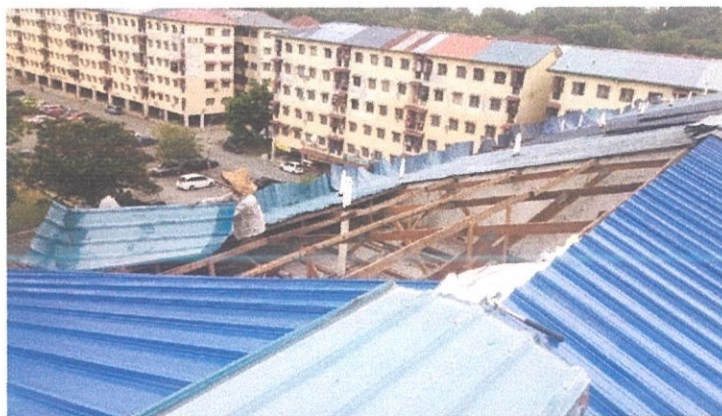
Figure 3.3: Dismantle of existing roof structure
