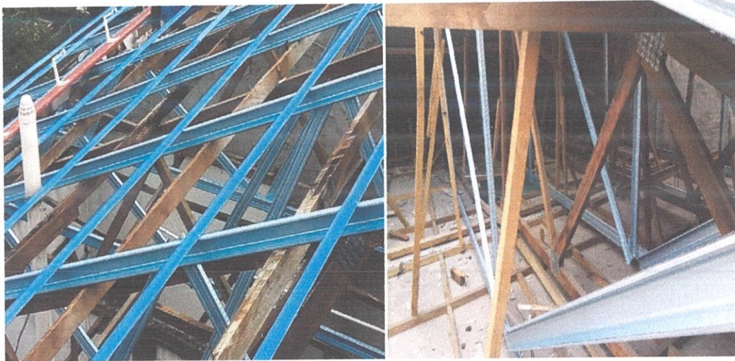
Figure 3.6: Installation of new trusses system
