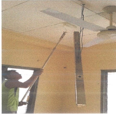
Figure 3.16: Apply ceiling finishes
