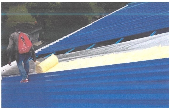
Figure 3.9: Installation of Fiber Glass Wool
