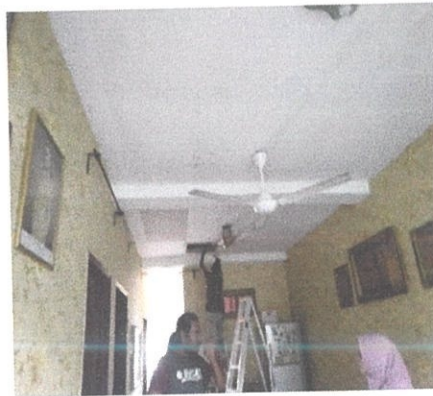
Figure 3.15: Installation of ceiling
