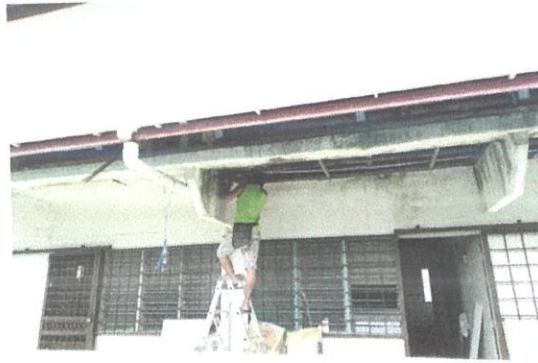
Figure 3.14: Installation of ceiling structure
