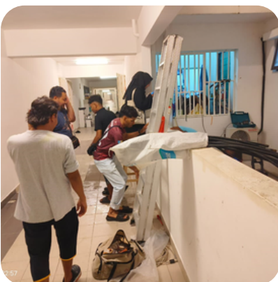
Resident's unit clogged piped - assist service provider unclog
