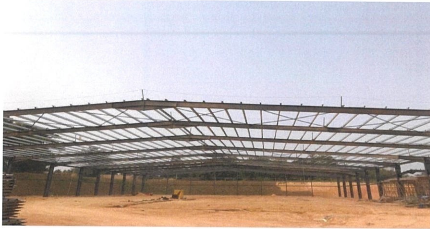
Figure 3.16: Bracing has been installed at lawn bowl
