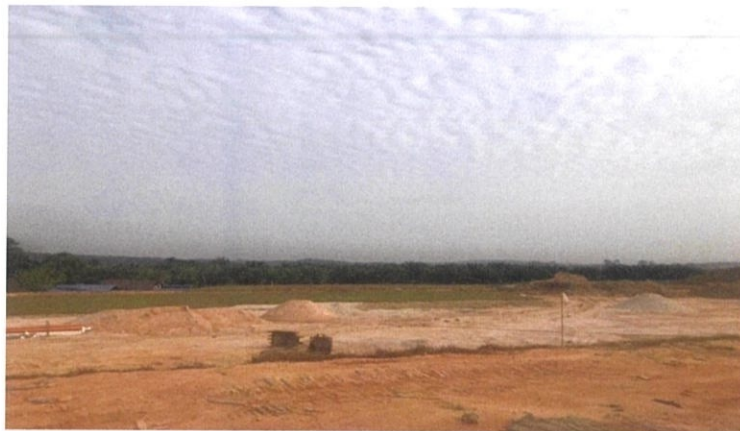
Figure 3.2: Process of site clearance
