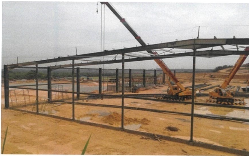
Figure 3.18: Installation work of purlin at lawn bowl
