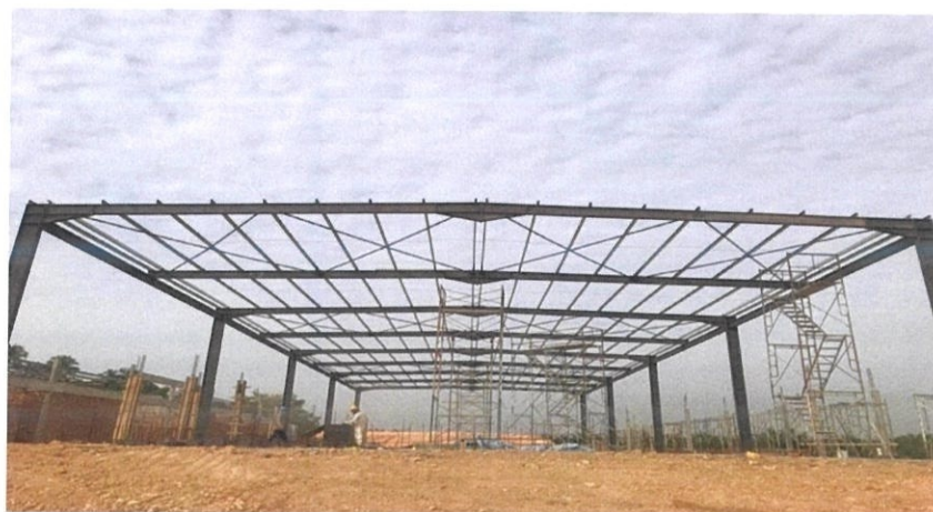
Figure 3.17: Bracing has been installed at main pavillion
