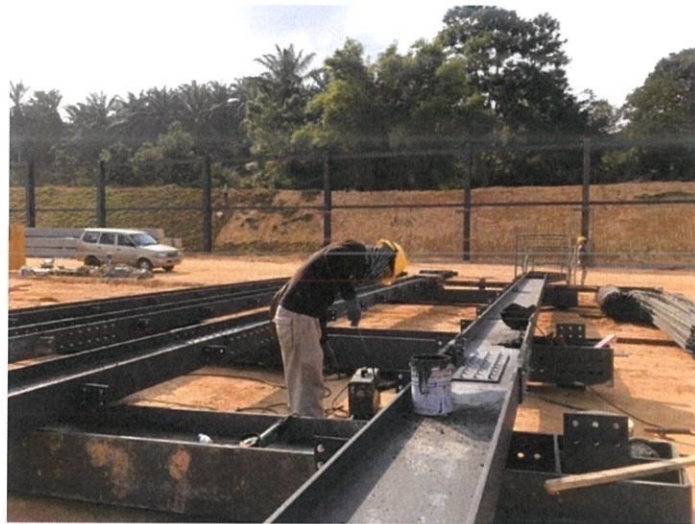
Figure 3.32: Worker is painting the steel to cover the faded colour
