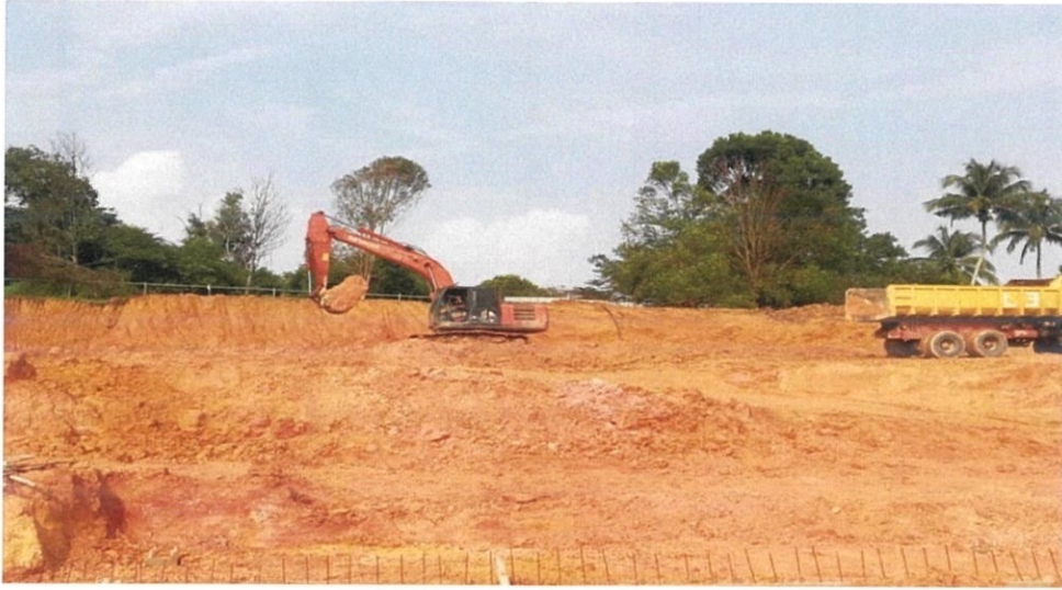
Figure 3.6: Excavation work at level 1m by using excavator
