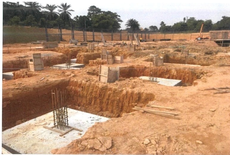
Figure 3.9: Concrete stump at level 1.2m
