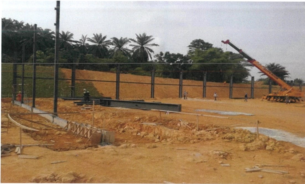
Figure 3.13: Installation work of tie-beam at lawn bowl
