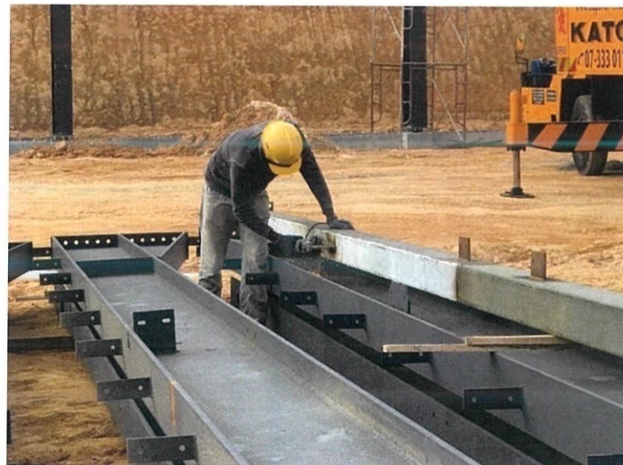
Figure 3.33: Worker is repairing the defect of steel
