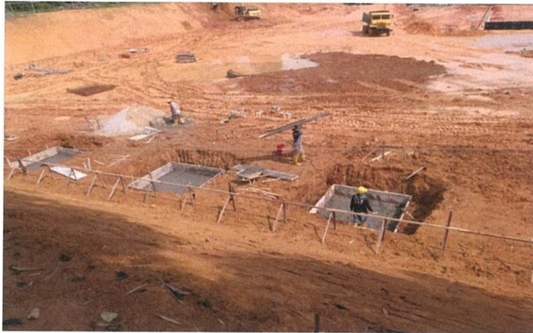
Figure 3.7: Concrete pad footing at level 1m
