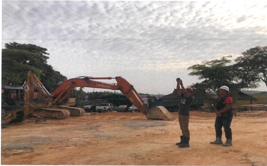
Figure 3.5: Site supervisor and safety officer monitoring the excavation work
