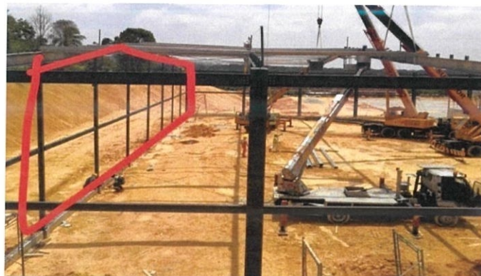
Figure 3.28: Unstructured column at lawn bowl
