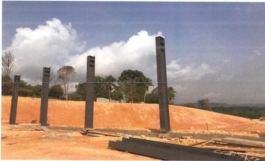
Figure 3.11: Installation work of lawn bowl column
