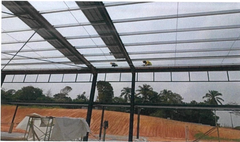
Figure 3.21: Installation work of roof gutter at lawn bowl
