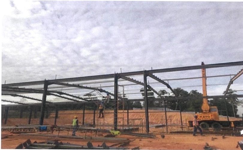
Figure 3.14: Installation work of portal frame at lawn bowl
