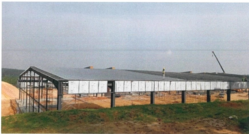
Figure 3.23: Progress installation of roof covering at petanque
