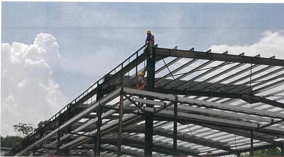
Figure 3.20: Progress installation of polycarbonate frame at lawn bowl and main pavillion
