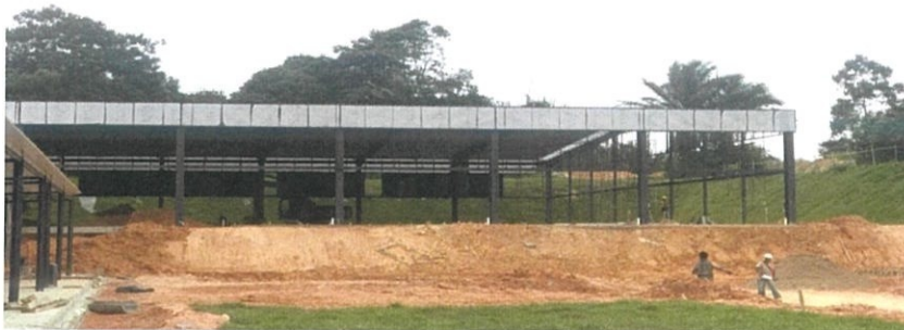
Figure 3.24: Progress installation of roof covering at lawn bowl
