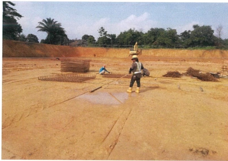
Figure 3.4: Leveling work at main pavillion
