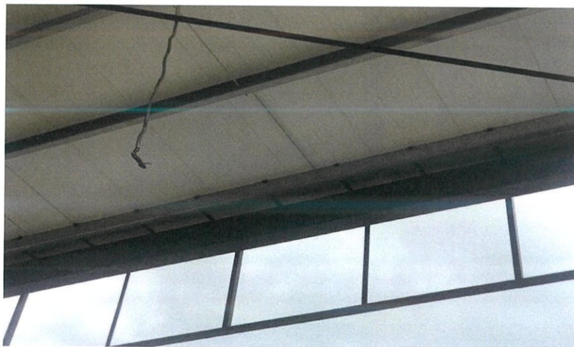
Figure 3.22: Roof gutter has been installed at petanque
