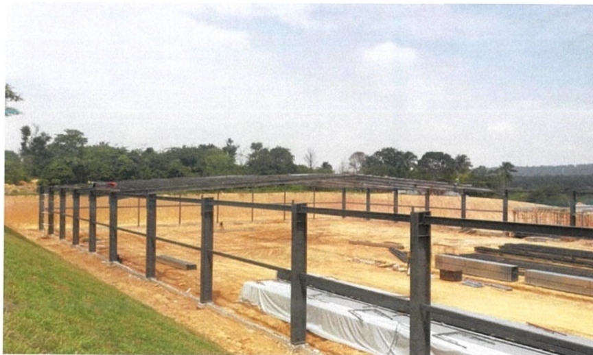
Figure 3.12: All column for lawn bowl has been installed
