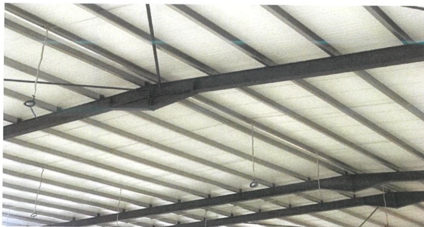
Figure 3.19: Purlin has been installed at main pavillion
