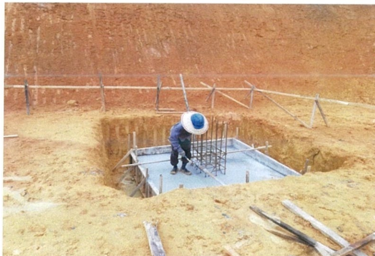
Figure 3.8: Worker measuring the level
