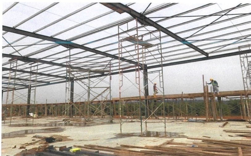
Figure 3.15: Portal frame has been installed at lawn bowl
