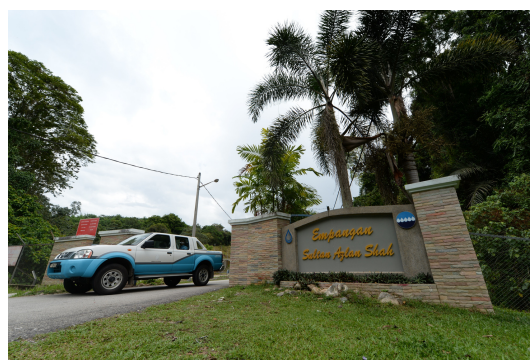
Figure 18: Sultan Azlan Shah Dam
