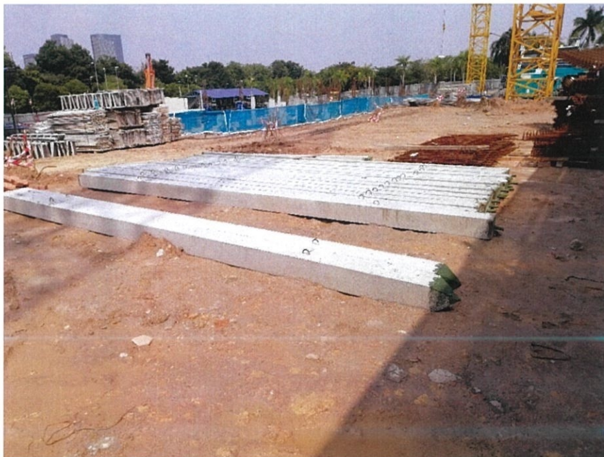
Figure 3.9: RC Pile
