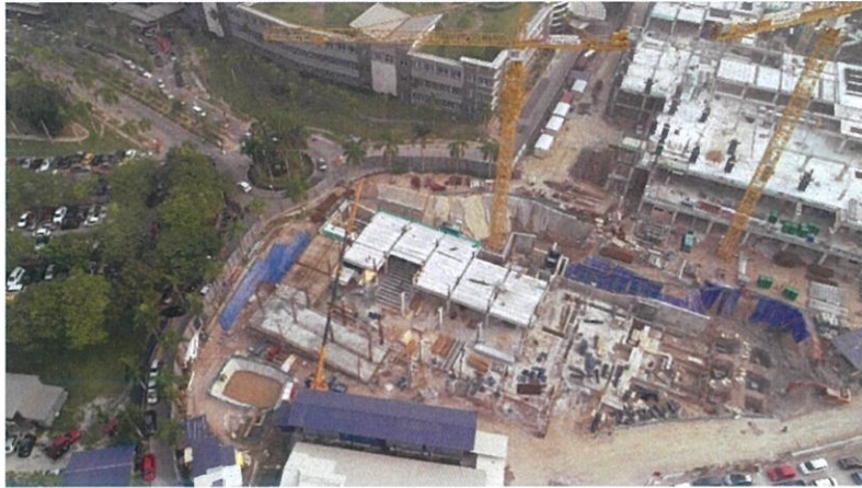
Figure 3.5: Sky view of multilevel car park by drone.
