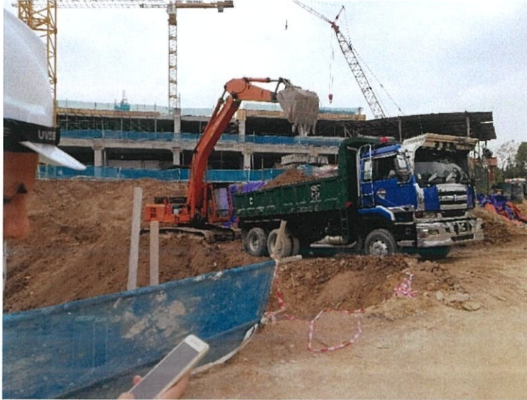
Figure 3.16: Excavate soil was loaded into dump truck by using excavator.
