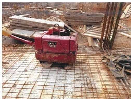
Figure 3.25: 1-Ton compactor
