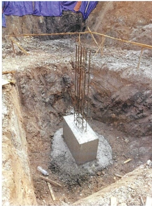
Figure 3.22: Result for concrete work for pile cap.
