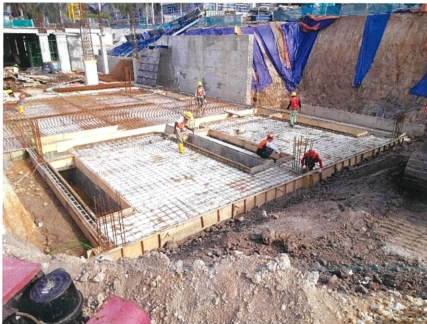
Figure 3.31: Reinforcement for ground slab
