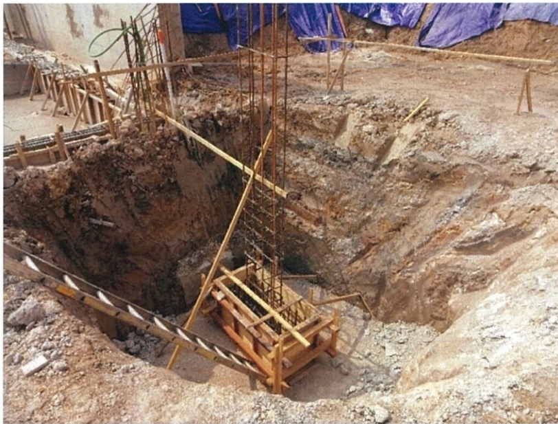
Figure 3.21: Reinforcement bar installation for pile cap
