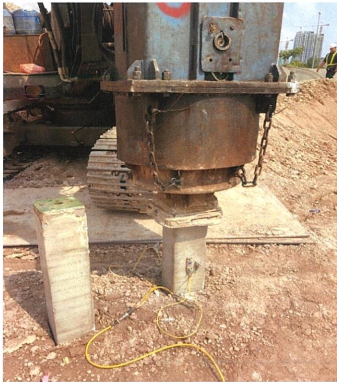
Figure 3.39: PDA test ongoing
