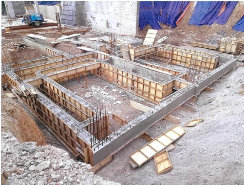
Figure 3.29: Ground beam after concrete done
