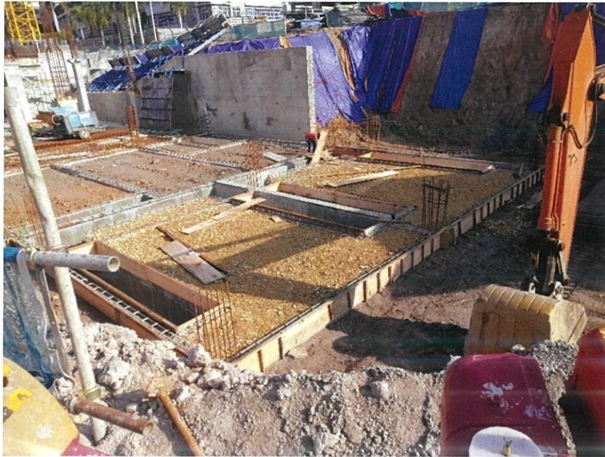
Figure 3.30: Formwork for ground slab
