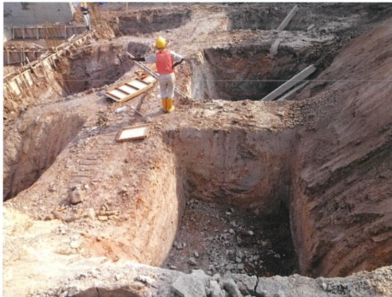
Figure 3.18: Cut off pile
