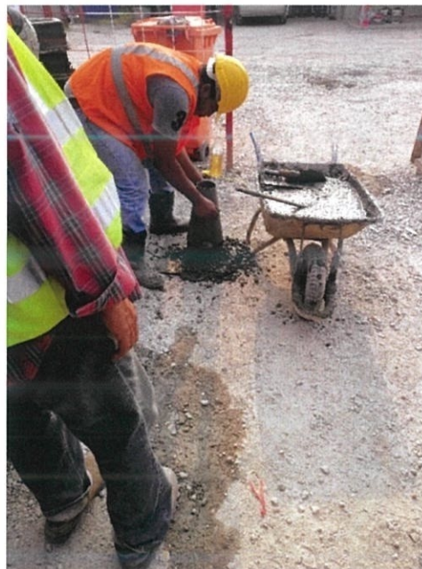
Figure 3.28: Slump test was done at the site
