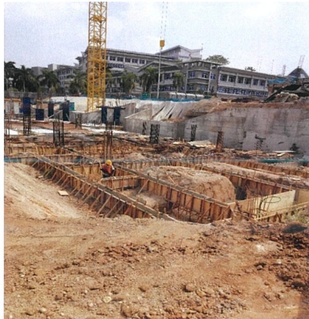
Figure 3.26: ground beam formwork
