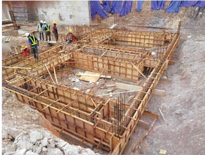
Figure 3.27: Reinforcement for ground beam
