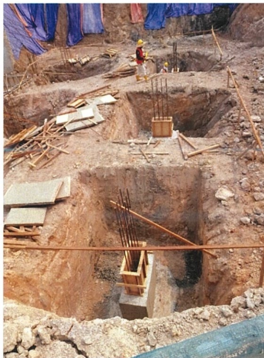
Figure 3.23: Formwork for stump
