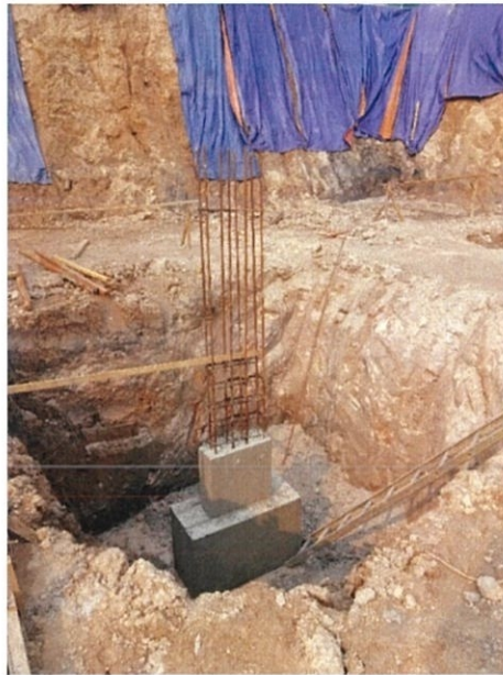
Figure 3.24: Result after concrete of stump
