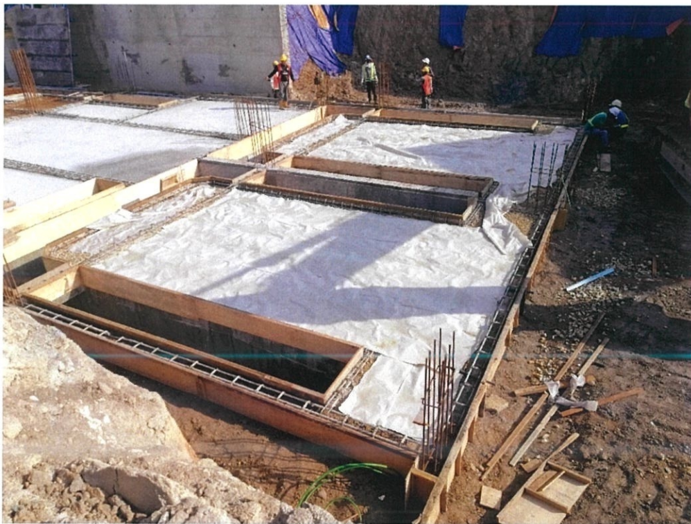
Figure 3.33: Damp-Proof Membrane (DPM)
