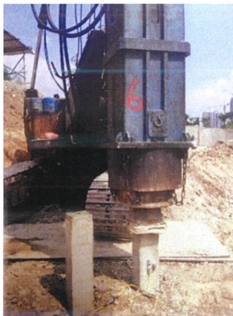
Figure 3.14: RC Pile was driven into foundation by using hydraulic hammer
