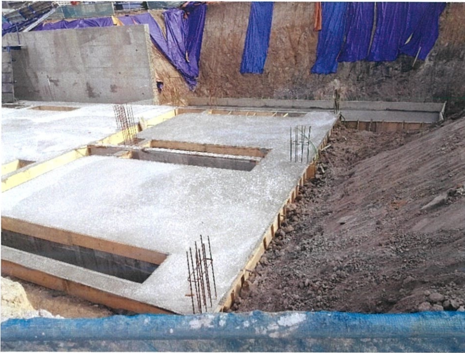
Figure 42: Ground slab was done concrete
