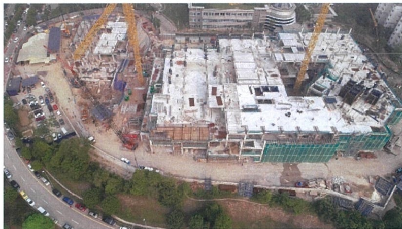
Figure 3.3: Sky view of site. (Source: Drone)
