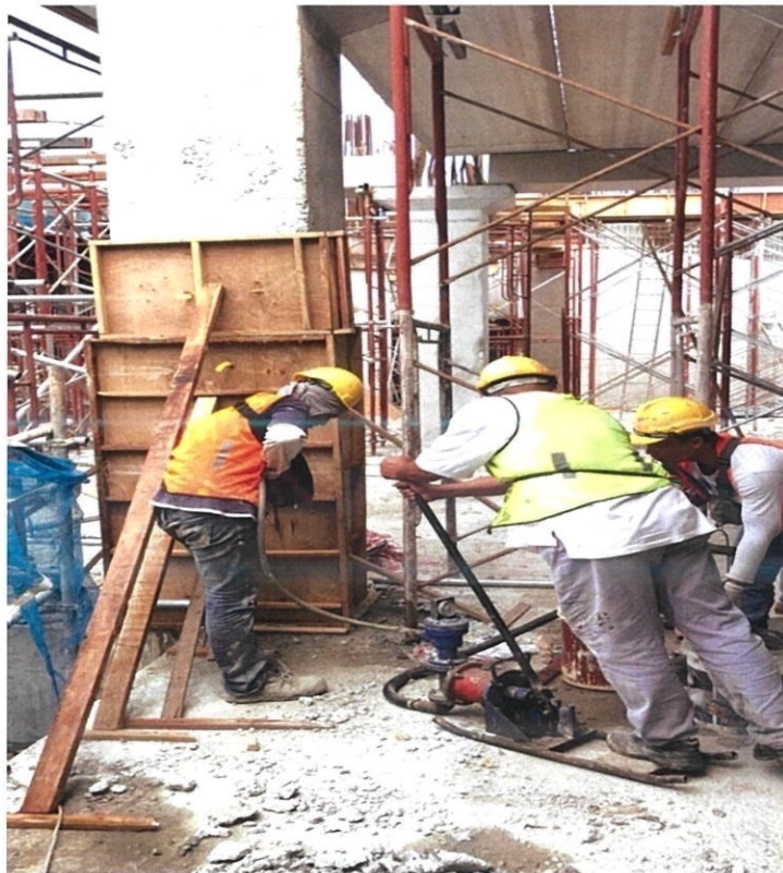
Figure 3.41: Pressure grouting test on going
