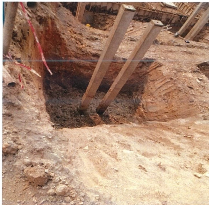
Figure 3.17: Open Cut excavation.
