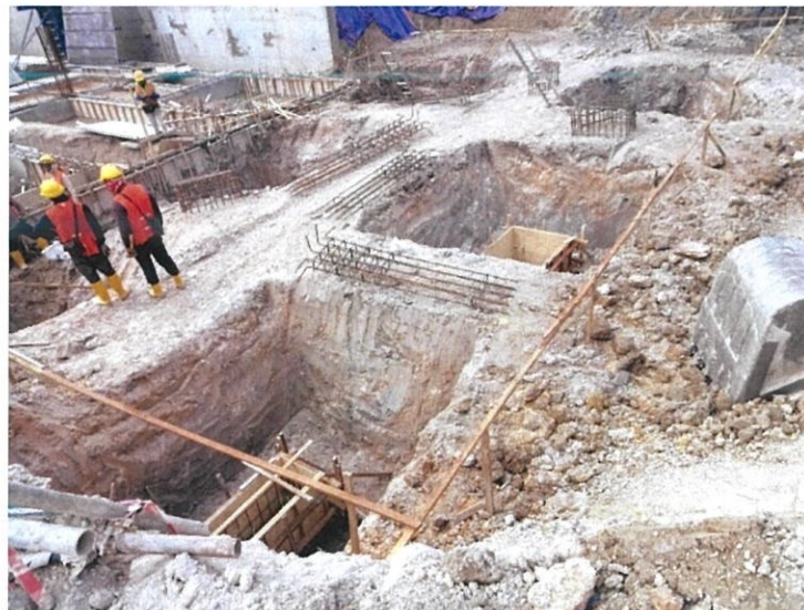
Figure 3.20: Formwork for pile cap
