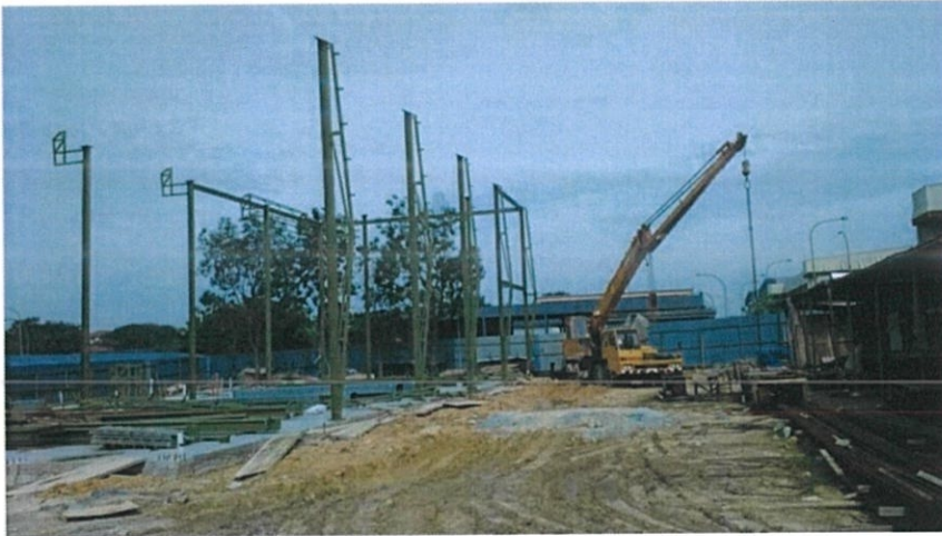
Photo 3.12: The workers are tighten the bolt and nut.
