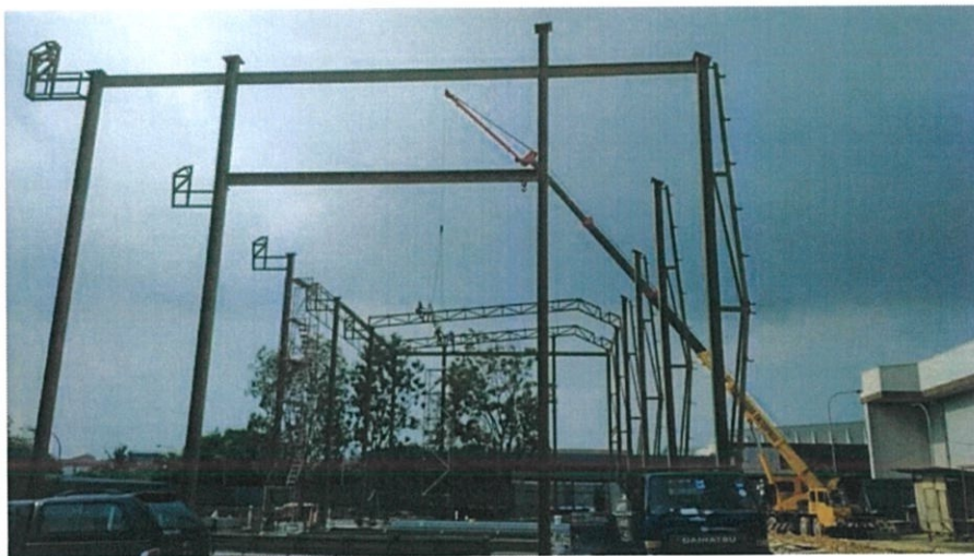
Photo 3.13: Shows the secondary beam was lifting by mobile crane.
