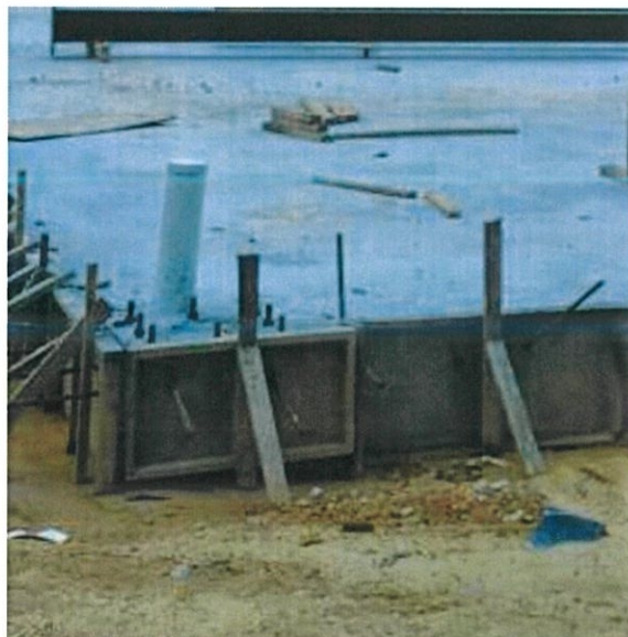
Photo 3.6: Shows the holding down rates are ready to receive materials.
