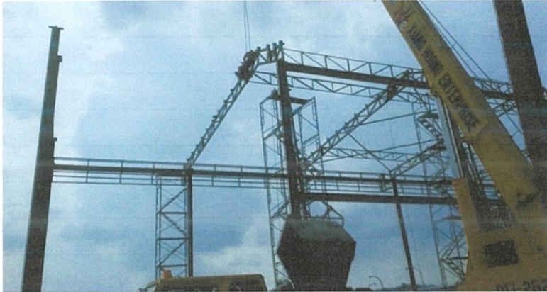
Photo 3.14: Shows the workers were doing fillet weld.
