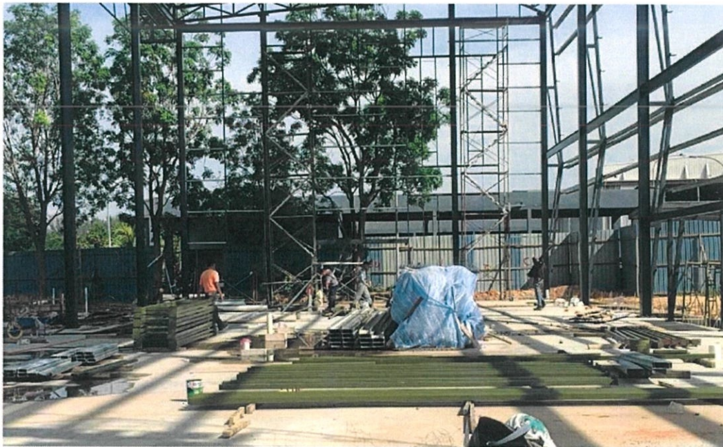
Photo 3.5: Shows the materials just placing on the site.
