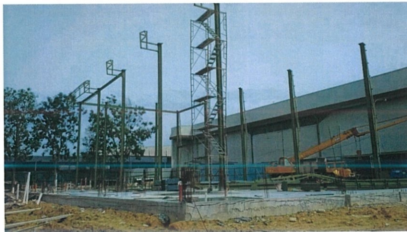
Photo 3.11: The mobile cranes were lifting by mobile cranes.
