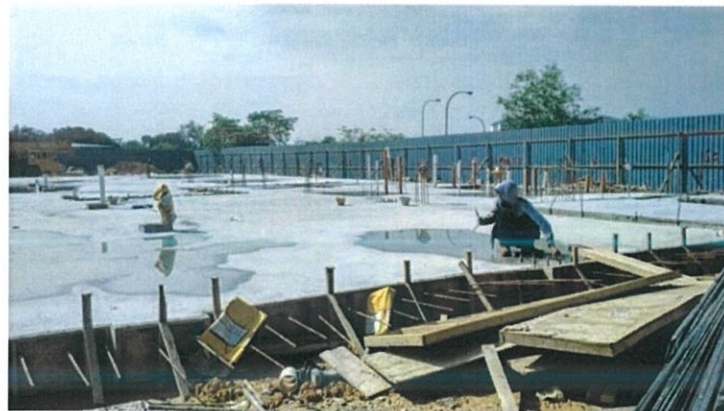
Photo 3.4: Show the holding down bolts completely install.
