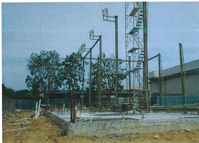
Photo 3.10: The all columns are completely install.
