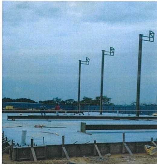
Photo 3.7: The I-beam are ready to install.
