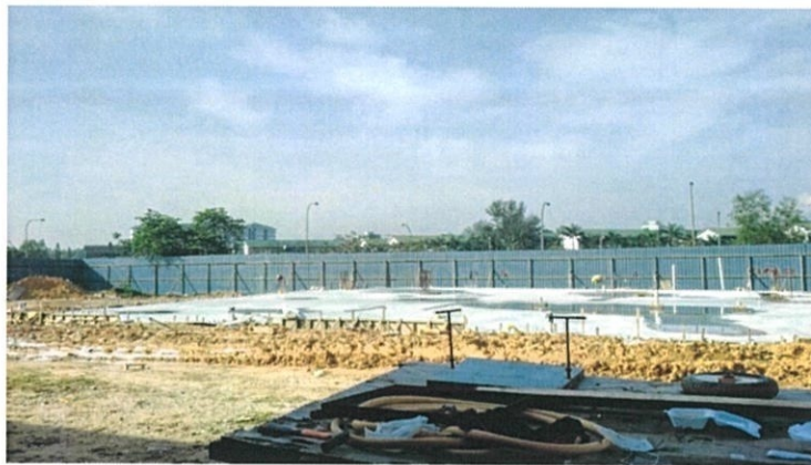
Photo 3.3: Shows the ground slab completely finish.
