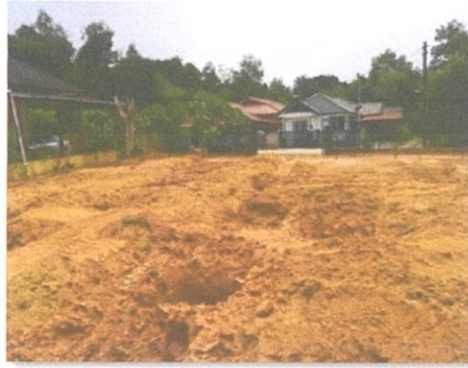
Photo 3.14 : the excavation of footing
