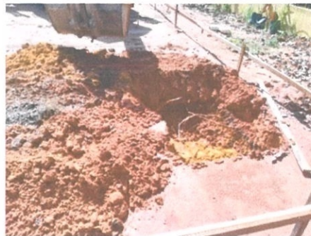
Photo 3.1: the clay soil at the site during excavation
