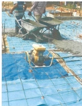
Photo 3.26 : the vibrator machine
