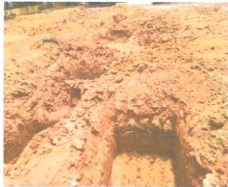
Photo 3.15: the depth of the footing is 3 feet
