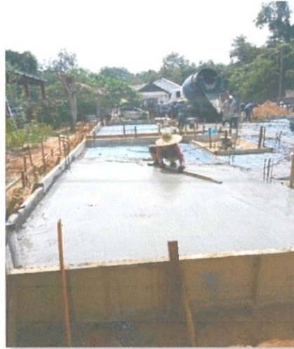
Photo 3.27 : the workers used wooden trowel to concrete to create flat surface
