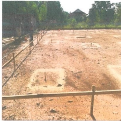
Photo 3.12: the position of footing was pegged
