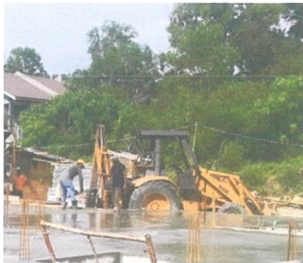
Photo 3.3 : the backhoe used for footing construction
