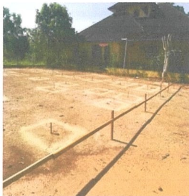
Photo 3.13: shows the location of the footing that has been marked
