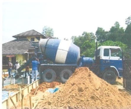
Photo 3.6: the truck mixer
