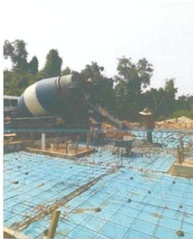
Photo 3.24 : the concrete was poured into a wheelbarrow
