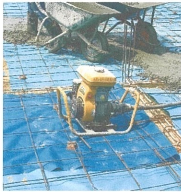
Photo 3.8: the vibrator used to compact the concrete.
