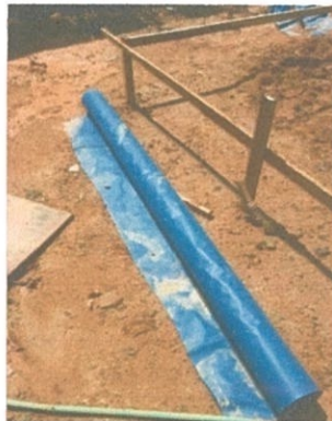
Photo 3.18 : the plastic membrane damp proofing
