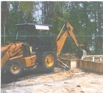
Photo 3.4: the backhoe used for excavated the soil
