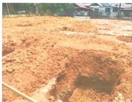
Photo 3.2: the size of pad footing at the site
