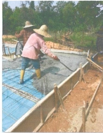
Photo 3.25 : the workers was compact the concrete using vibrator
