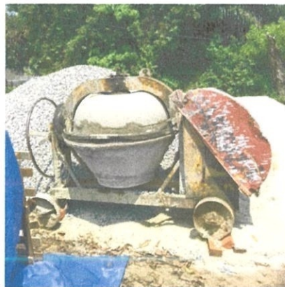
Photo 3.5: the concrete mixer at the site
