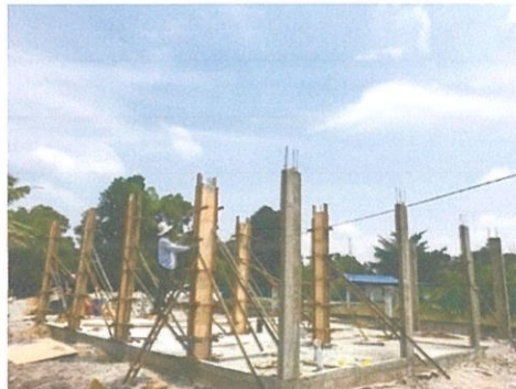
Photo 3.29 : the column starter bars was erected
