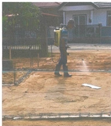
Photo 3.21: the workers was applied the anti termite to the ground
