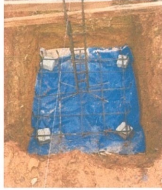
Photo 3.19: the brc and stump were place into the footing
