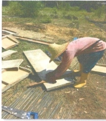
Photo 3.17: the workers was measured the length of formwork
