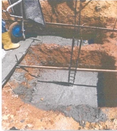
Photo 3.20: a layer of concrete was set
