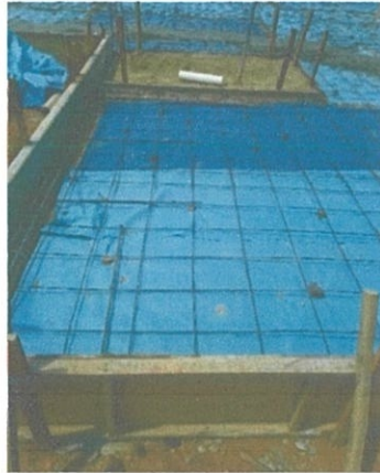
Photo 3.23: the waterproofing and the brc reinforcement
