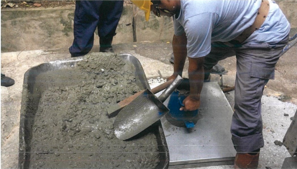
Figure 3.8: Lift the mould vertically
