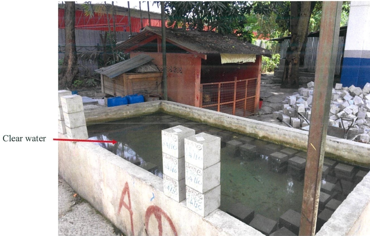
Figure 3.12: Curing in clear fresh water
