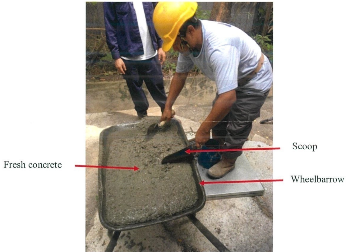
Figure 3.7: Fill the slump
