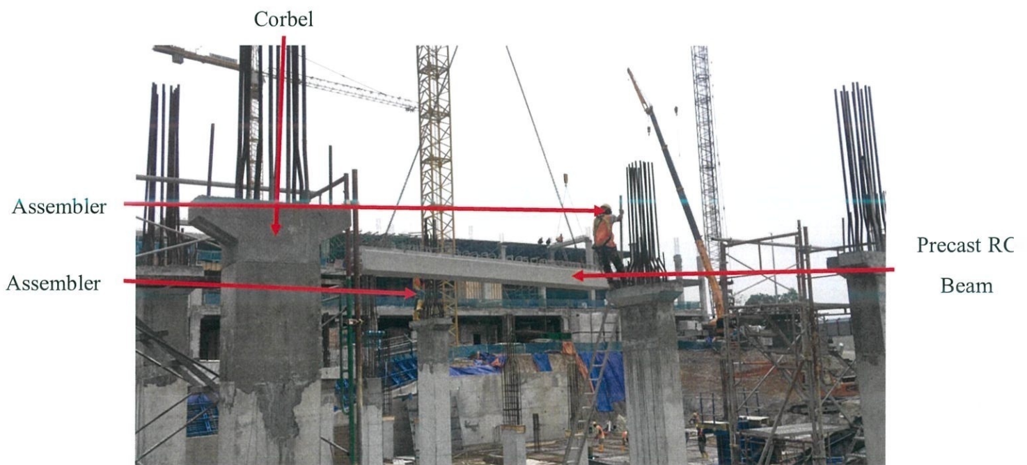
Figure 3.16: The installation of precast RC beam
