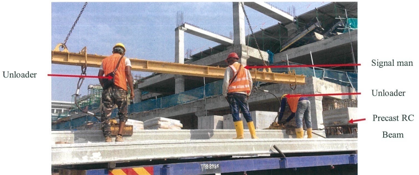
Figure 3.14: Unloading IBS
