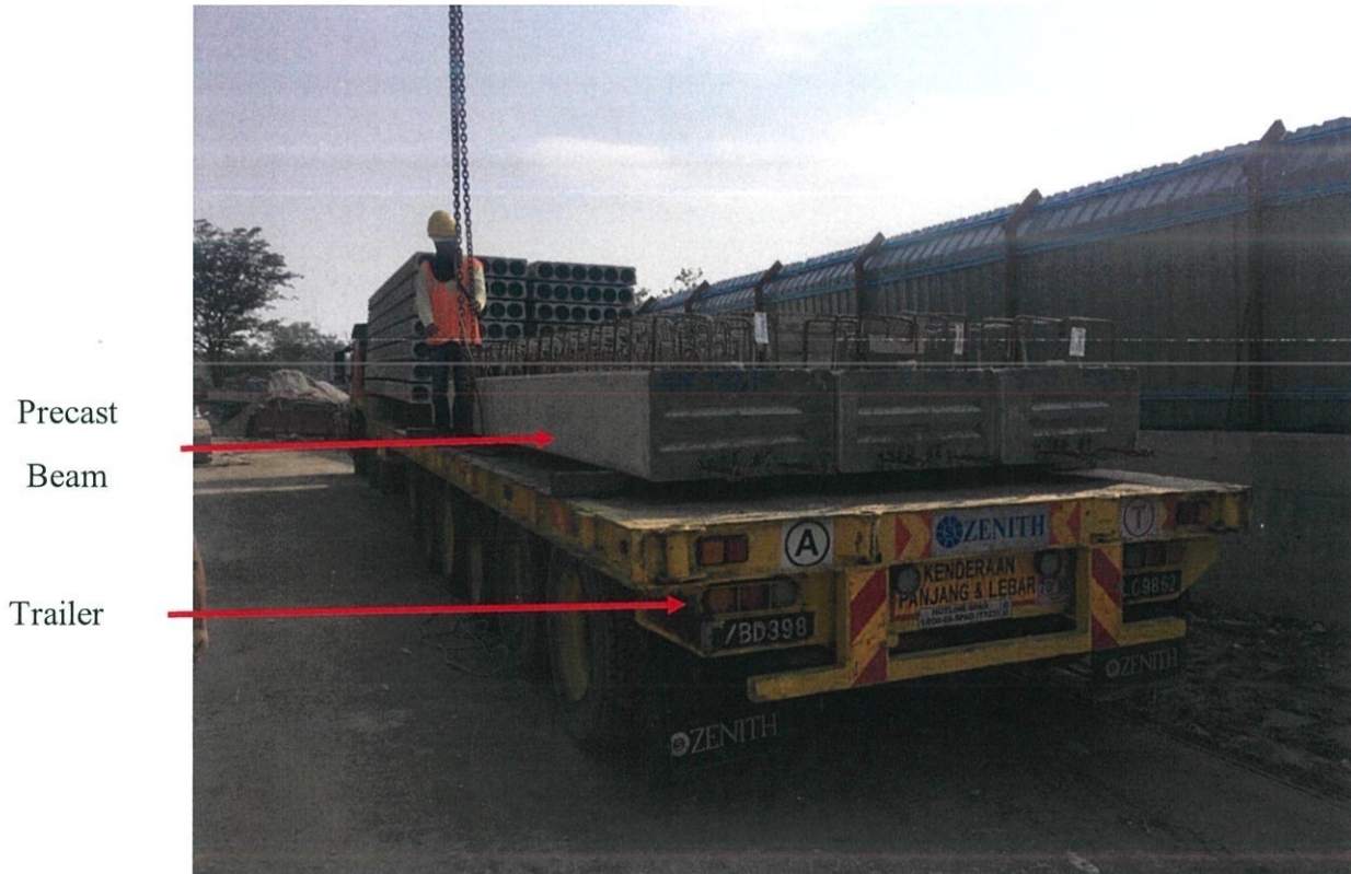
Figure 3.13: The precast beam was load on trailer
