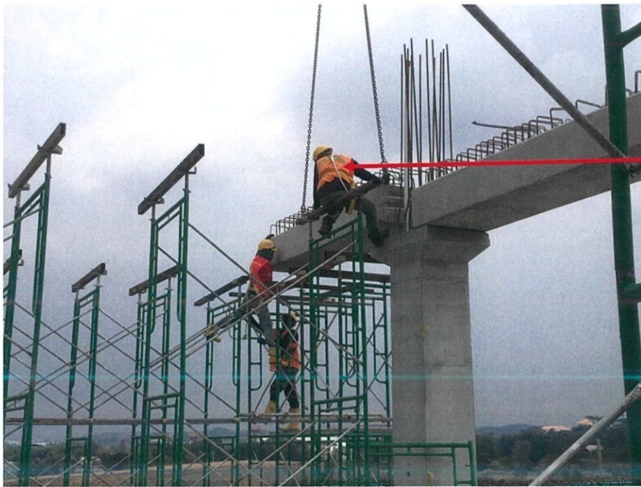
Figure 3.18: Installer guide the beam placed into position
