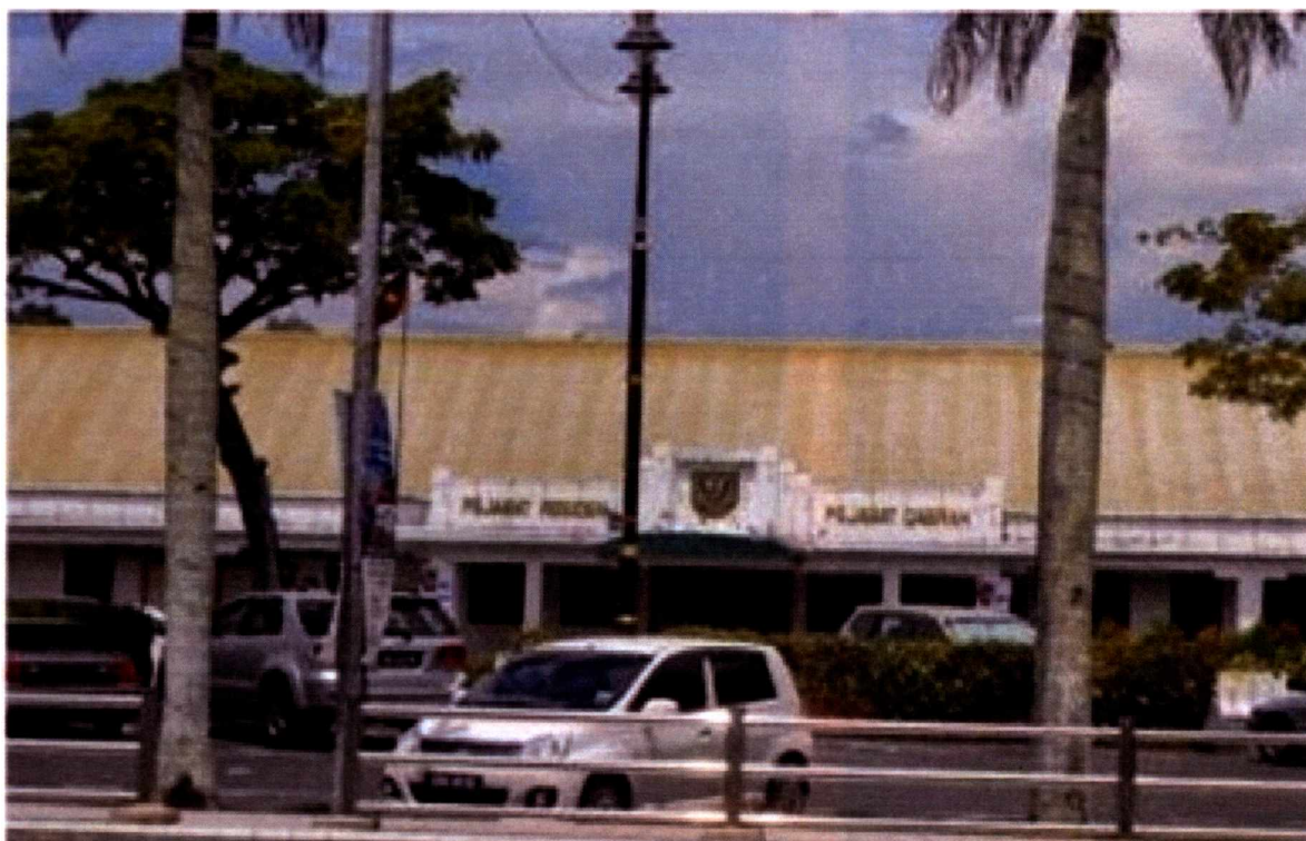
Picture1.2: Miri Resident Office
