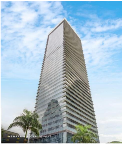
Figure 4: Menara AIA CapSquare
