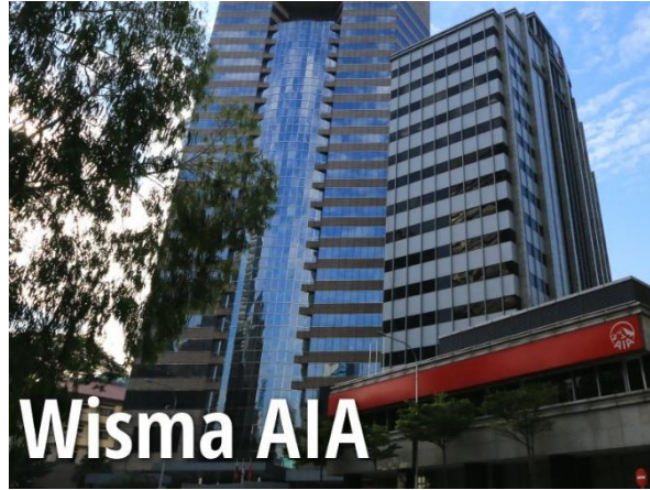
Figure 5: Wisma AIA Customer Center
