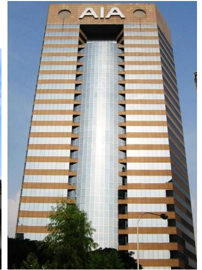
Figure 6: Menara AIA Malaysia's Headquarter
