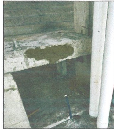
Figure 3.23 Recover the spalling concrete
