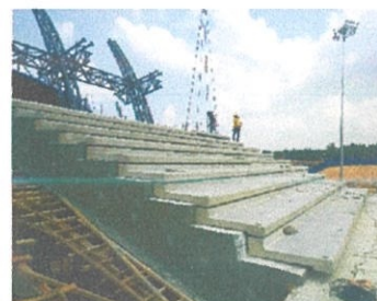
Figure 1.7 The precast concrete for seating area is installed
