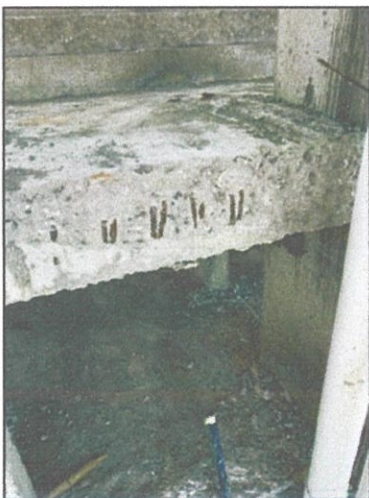
Figure 3.22 Spalling concrete
