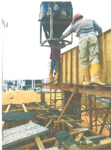
Figure 3.12. The concreter is pouring concrete
