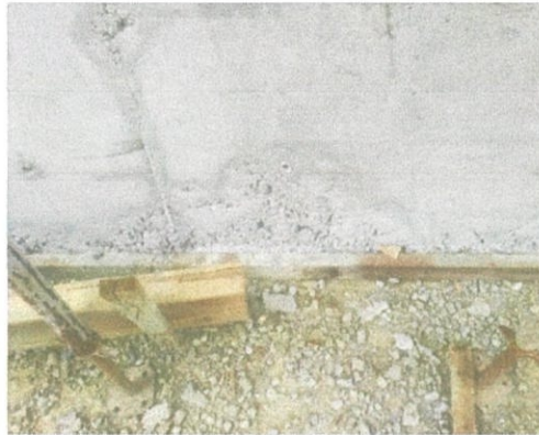
Figure 3.20 Honeycomb defect
