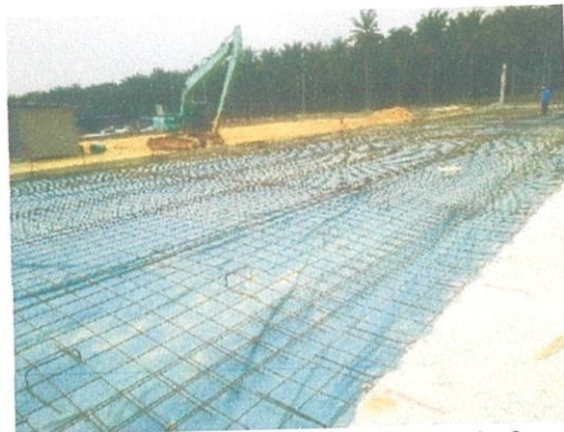
Figure 3.19 Surface should be clean before concreting
