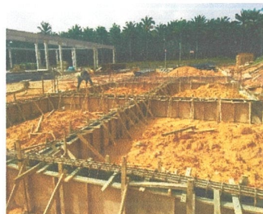
Figure 3.17 Installation of bar at ground beam
