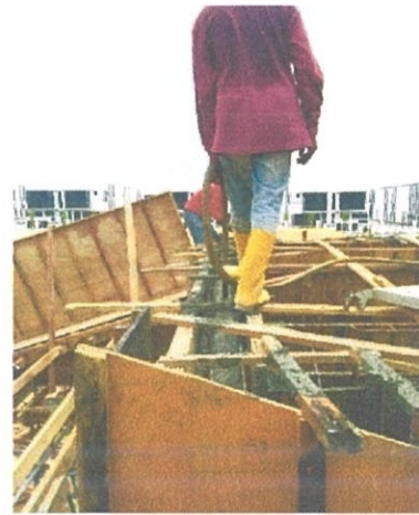
Figure 3.13 The concreter is compacting the poured concrete
