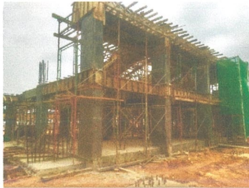
Figure 3.16 Formwork of beam
