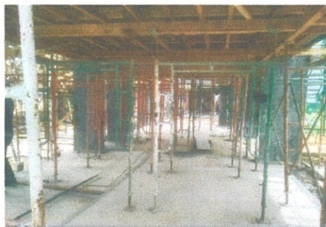
Figure 3.8 Scaffold to support formwork
