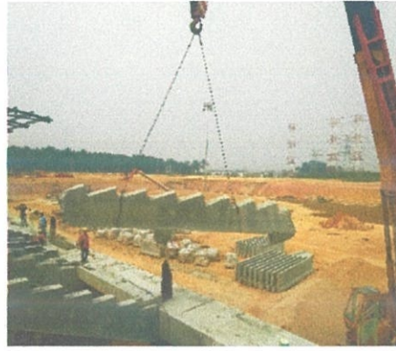
Figure 3.26 Removing the unacceptable slanting beam
