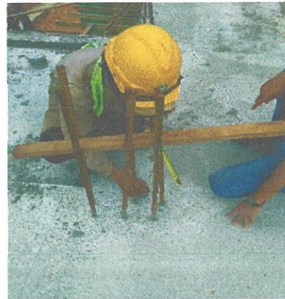
Figure 3.15 Setting out line mark
