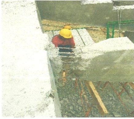
Figure 3.25 Cutting the connection bar
