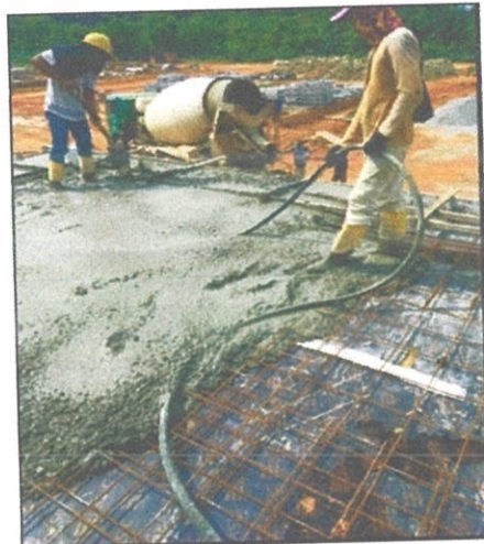
Figure 3.18 Compacting fresh concrete for slab
