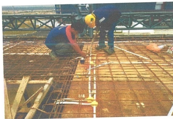
Figure 3.11 Installation of electrical conduit pipe
