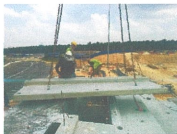
Figure 1.6 The installing work of precast concrete at seating area
