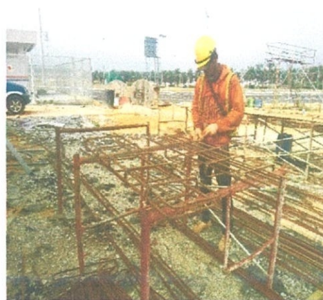
Figure 3.9. Fixing the BRC
