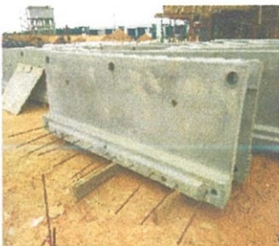
Figure 1.5 The precast concrete of seating area
