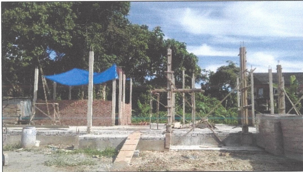
Figure 3.20: Site Condition Throughout The Delays
