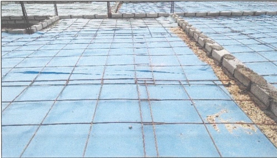
Figure 3.10: Overlapped Wiremesh
