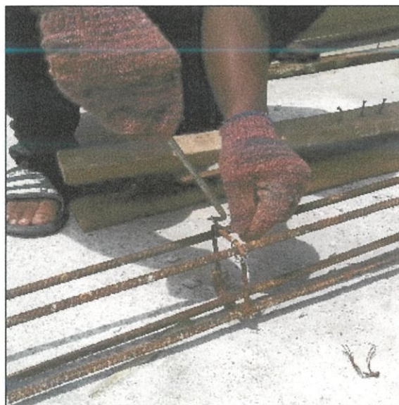
Figure 3.14: Fixing Reinforcement Bar
