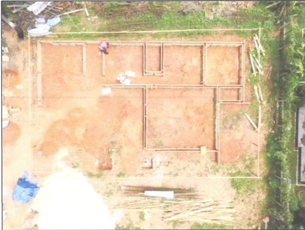
Figure 3.3: Top View of The Site During Formwork Installation
