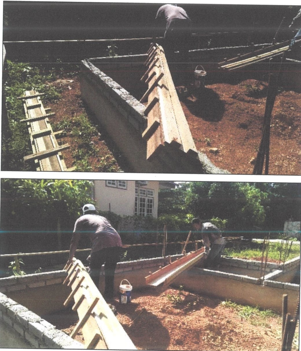
Figure 3.16: Assembling Work of Formworks
