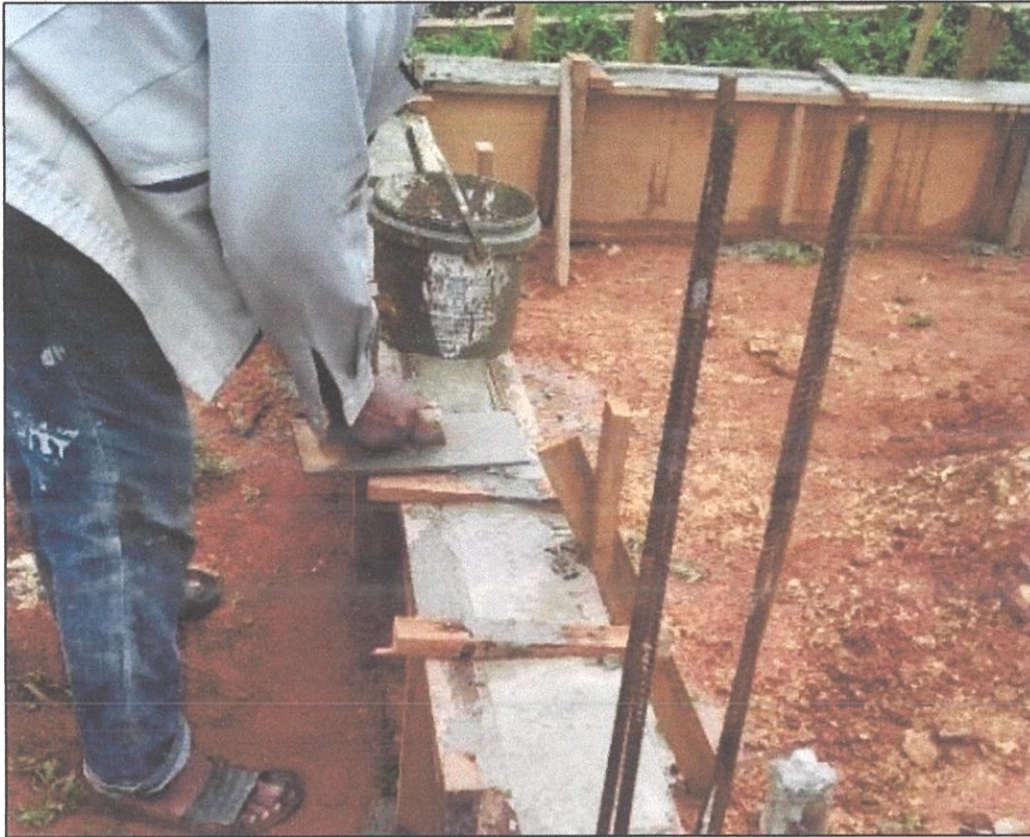
Figure 3.6: Concrete is Flattened on the Surface
