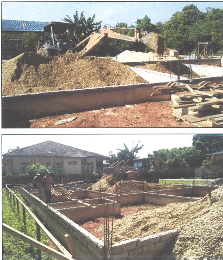
Figure 3.7: Sand Filling in The Slab Area
