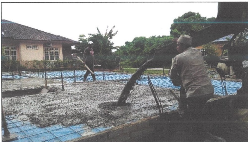
Figure 3.11: Concrete Pouring for Slab
