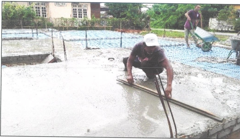
Figure 3.12: Concrete Spreading
