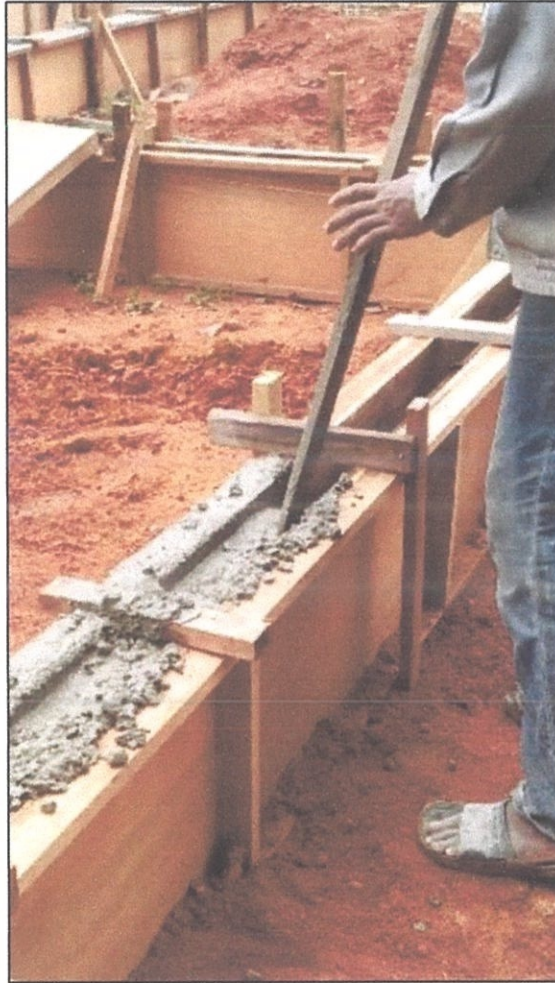
Figure 3.5: Concrete is Compacted
