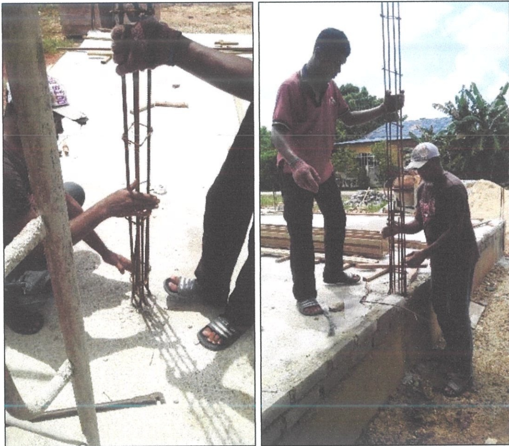
Figure 3.15: Reinforcement Bar Installation
