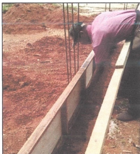
Figure 3.2: Formwork Installation for Ground Beam
