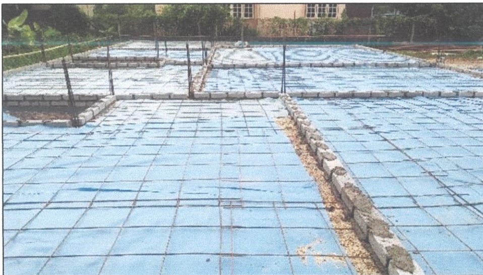
Figure 3.8: Plastic Barrier Installed Under Wiremesh
