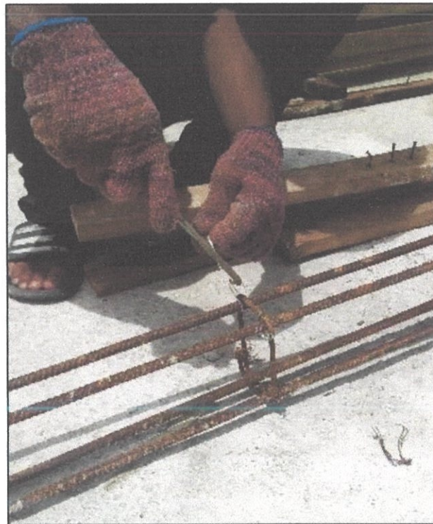
Figure 3.21: Fixing Reinforcement Bar for Column
