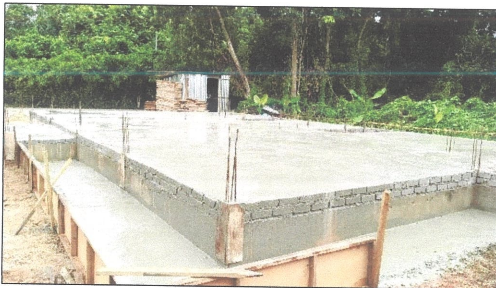
Figure 3.13: Curing Process of Concrete
