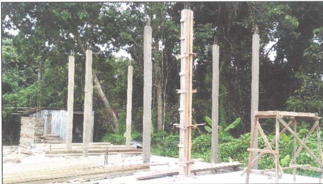
Figure 3.18: Column After Removing The Formwork
