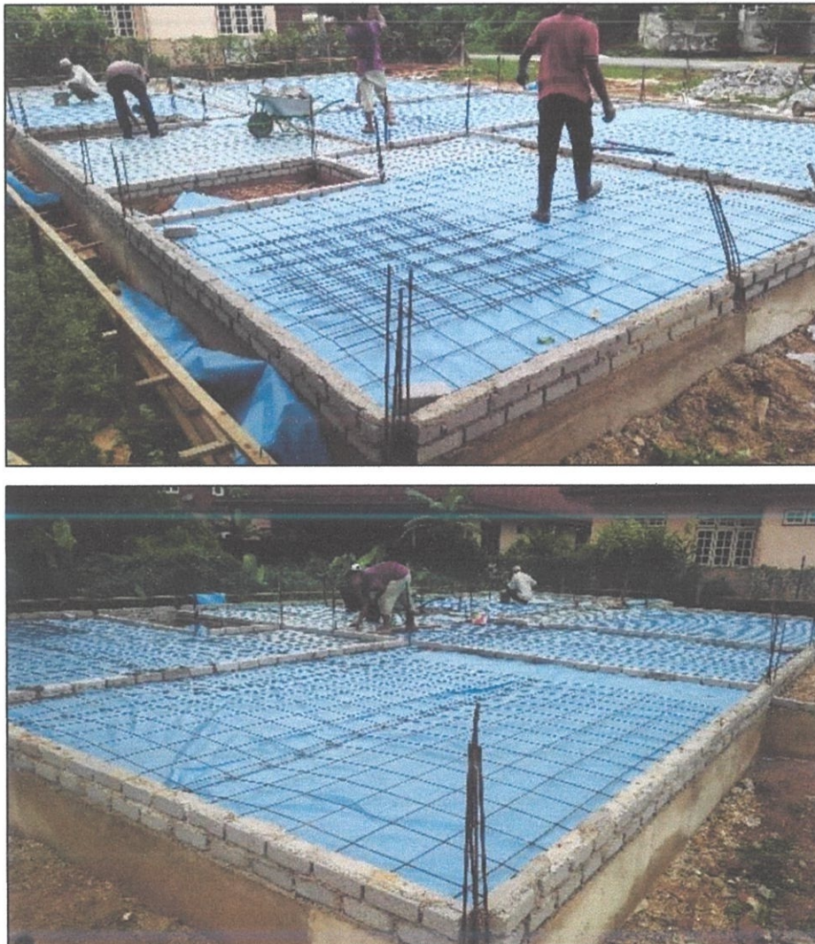
Figure 3.9: Wiremesh Installation
