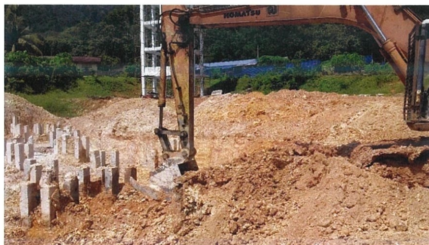
Figure 2.4.2.1 Excavation works to construct quarter
