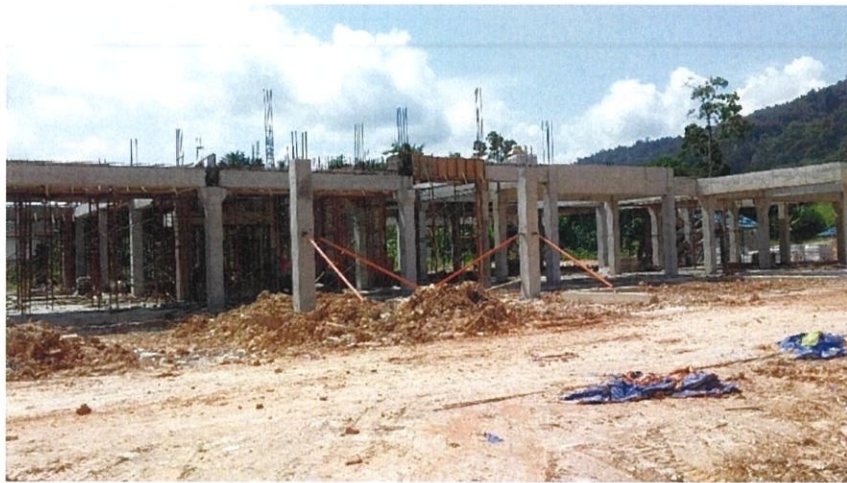
Figure 2.4.2 View of construction of clinic
