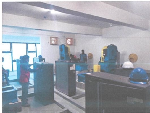
Figure 3.5 Lift motor room
