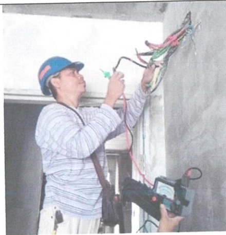
Figure 3.26 Meggar test
