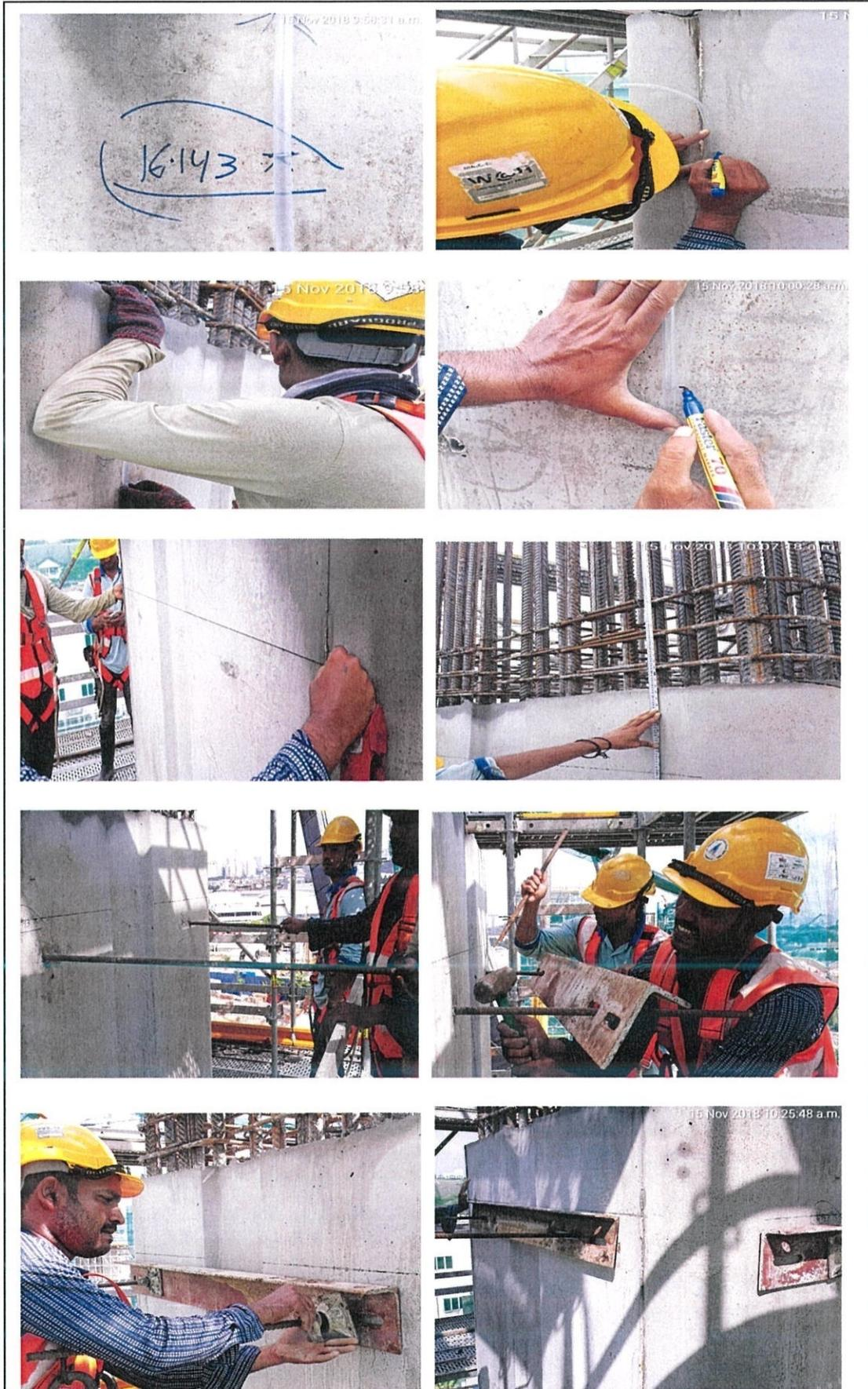
**Figure 3.2.20: The step by step of installing the stand jack by BCSC workers.**
