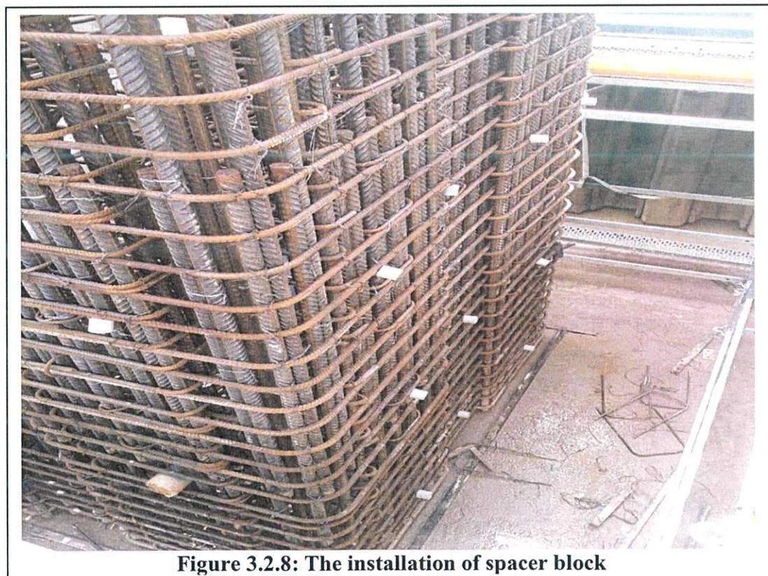
Upon completion of reinforcement bar installation, a joint inspection were carried out with SC to ensure reinforcement bars are installed according the IFC/construction drawing as well as the accordance of spacer block.
