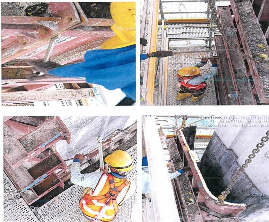
**Figures 3.2.16: The step by step of formwork removal.**
