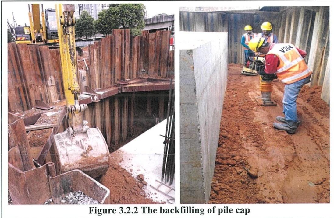
**Figure 3.2.2 The backfilling of pile cap**
