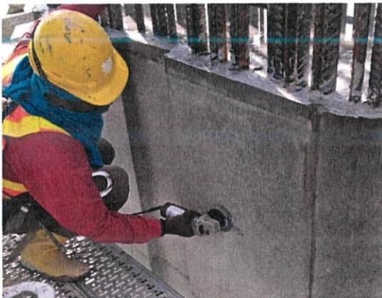
**Figure 3.3.5: The Pressure Grout Works by using Sika Grout 215**
