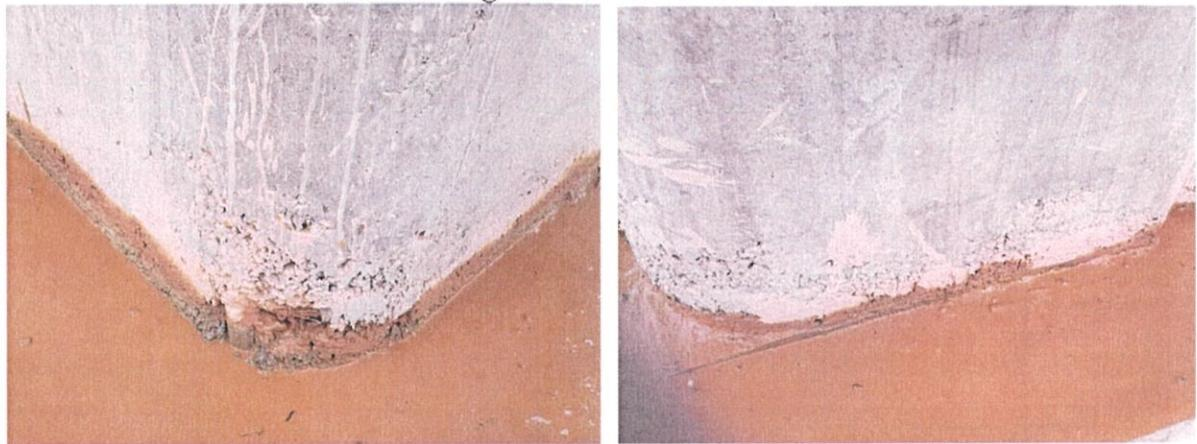
**Figure 3.3.2: A localized honeycomb at first casting pier column top of pile cap from NCR605 issued on 13<sup>th</sup> July 2018.**
