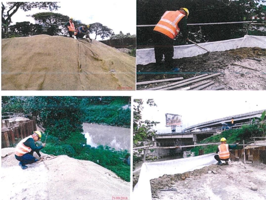
**Figure 3.4.2: The details of action taken that the sand slope has been protected with ECB**
