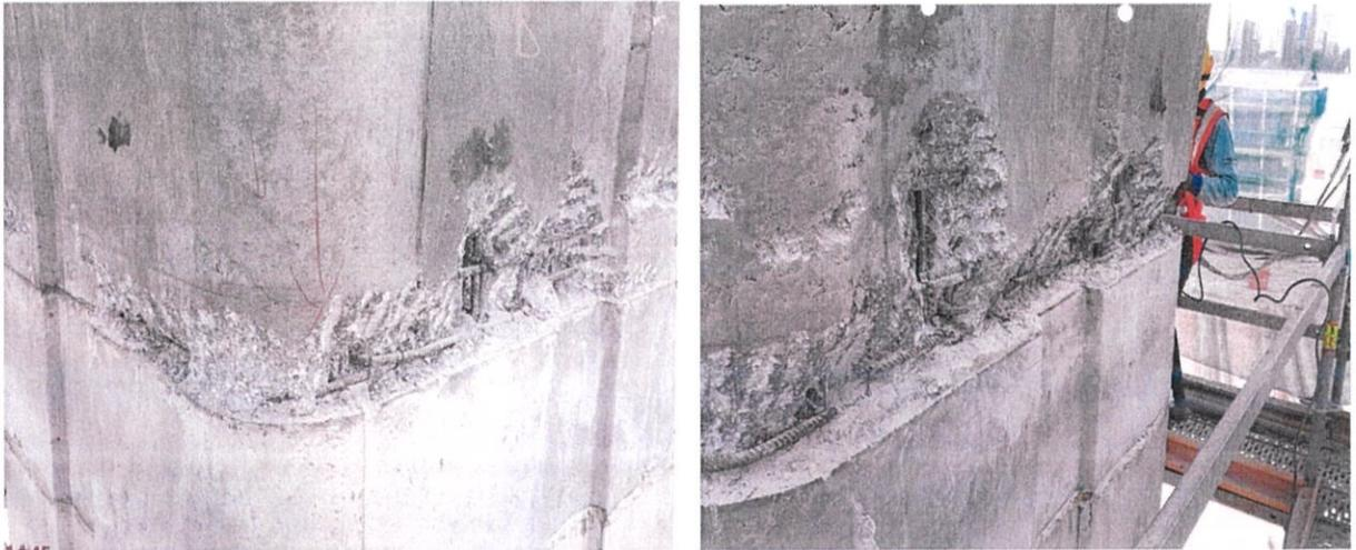
**Figure 3.3.1: A localized severe honeycomb at pier column and pier head construction joint at TNEN15 Kampung Malaysia. The root cause is insufficient of vibration during concreting works. This is NCR-00679**
