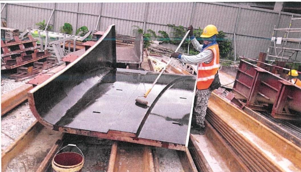
**Figure 3.2.10: The applicable of mould oil**
