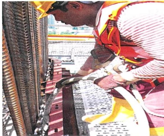
**Figure 3.2.15: The vibration works**
