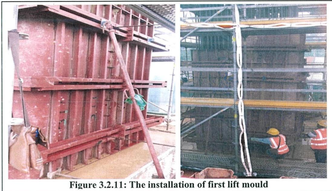
Joint survey for the column formwork as-built at the 4 corners were carried out. When necessary, chain block might be used for minor or fine tuning of mould alignment.
