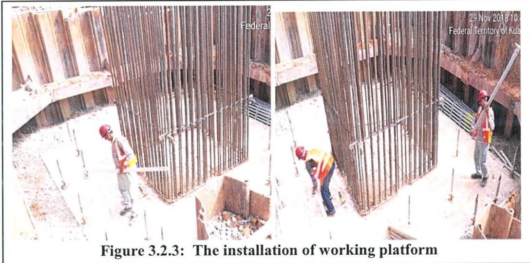
The reinforcement bars which are the starter bar and links were installed and lapped at locations where the starter bars for pier were installed earlier in the pile cap. The numbers, sizes and lengths and positions of all reinforcing bars, links, stirrups, spacer bars and other parts other steel reinforcement were installed in accordance with the IFC/Construction Drawings and specifications.
