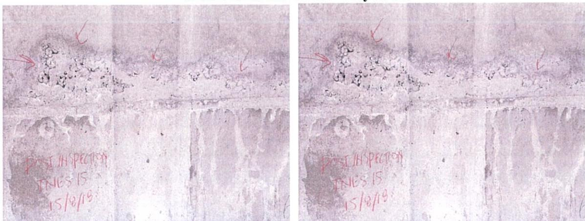
**Figure 3.3.3: NCR-00680 was issued on 20<sup>th</sup> August 2018 about a localized honeycomb pier at the third lift construction joint and just above the pile cap.**
