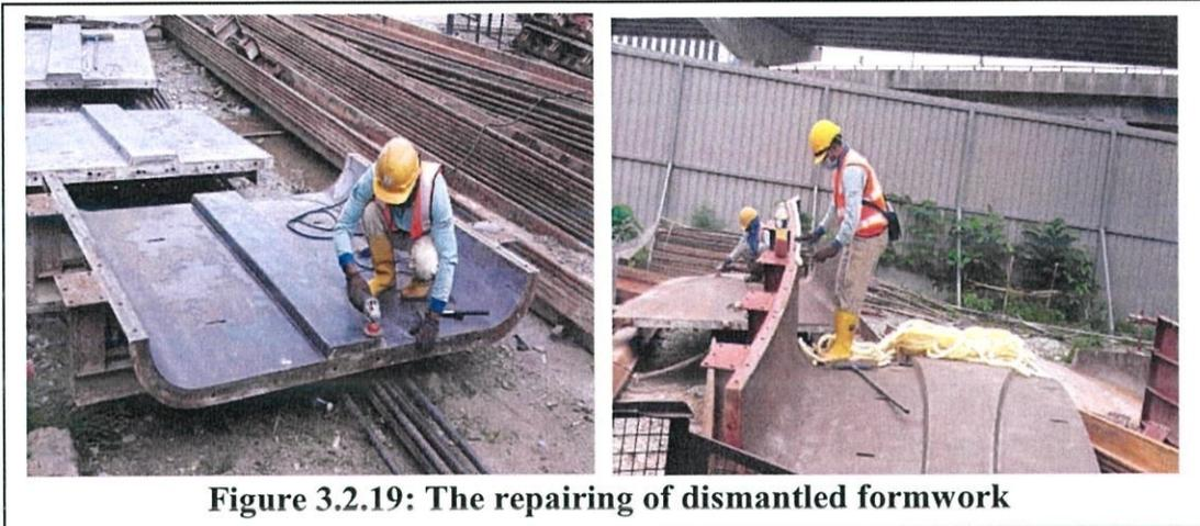
**Figure 3.2.19: The repairing of dismantled formwork**
